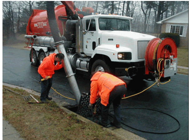
Storm drain cleaning. Photo: Ann Arundel County, Maryland.
