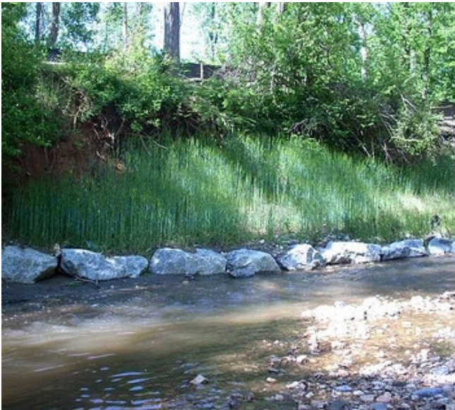
Stone toe protection, which prevents streambank erosion and shoreline erosion. Photo: Montgomery County, Maryland.
