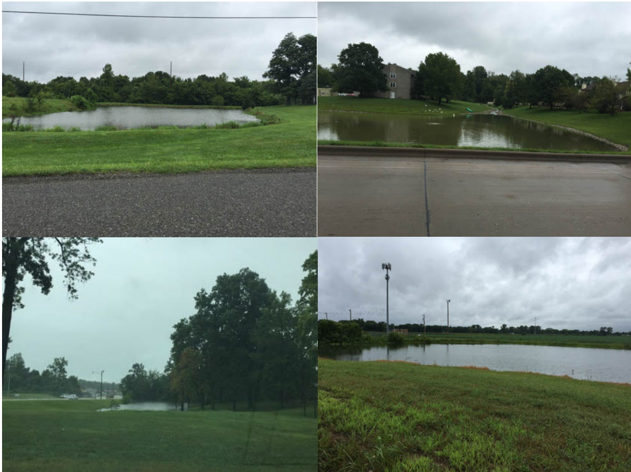
Figure A.42: Images from four detention basins from site visits on August 15, 2016. Note that Madison experienced precipitation for the past 24 hours and a flash flood warning was issued.
