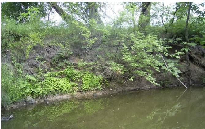
Isolated streambank erosion along Reach FC02 between Kelsey Road and Flint Lake
