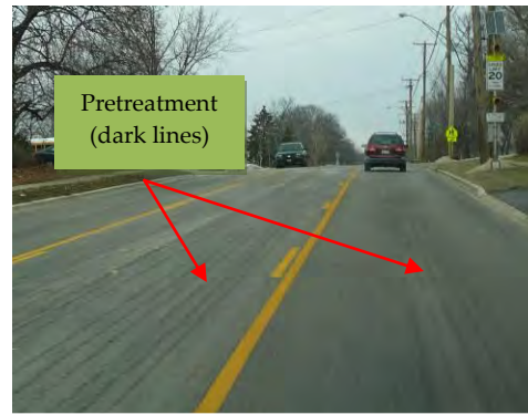
Figure 3-7. Pretreatment on Cedar Road, New Lenox
