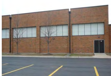
Figure 4-32. Roof Drains on Northeastern Side of School
