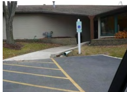
Figure 4-29. Entrance to New Lenox Park District Building
