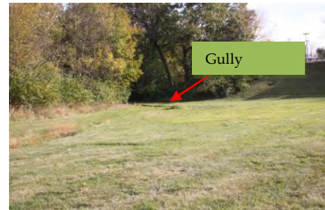
Figure 4-26. Silver Cross Hospital Regional Basin
