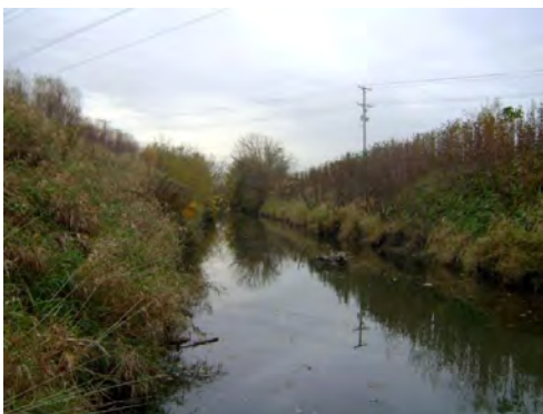
Figure 4-44. Union Ditch at 191 st Street, Tinley Park
