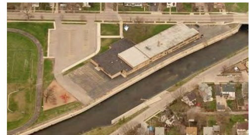
Figure 4-33. Aerial of School
