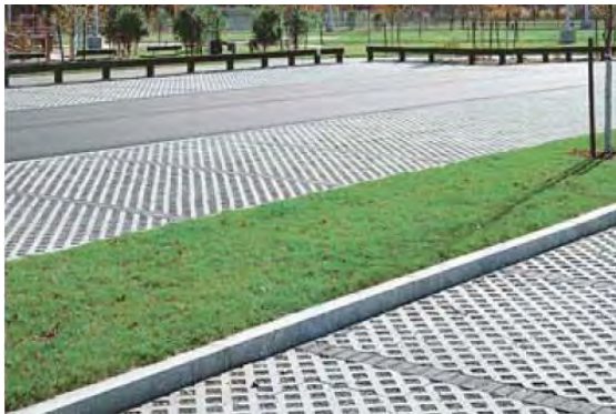
Figure 4-9. Concrete Grid Paver with Gravel Fill
