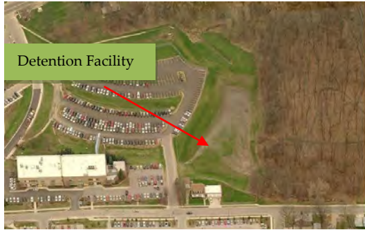
Figure 4-25. Silver Cross Hospital Regional Basin
