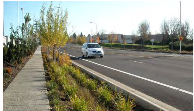
Figure 3-6. Arterial Roadway with Vegetated Swale and Porous Pavement Sidewalk
