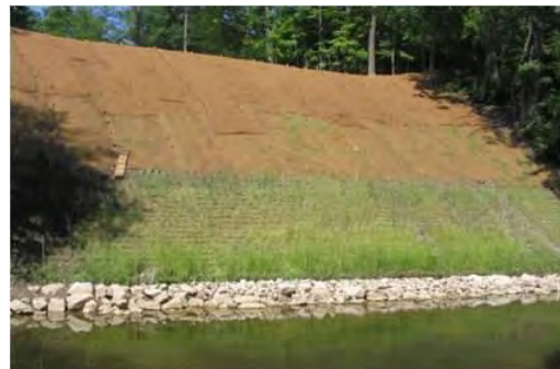
Figure 4-38. Rock Toe Protection with Geocells, Milwaukee, WI (Source: Inter-Fluve, Inc.)
