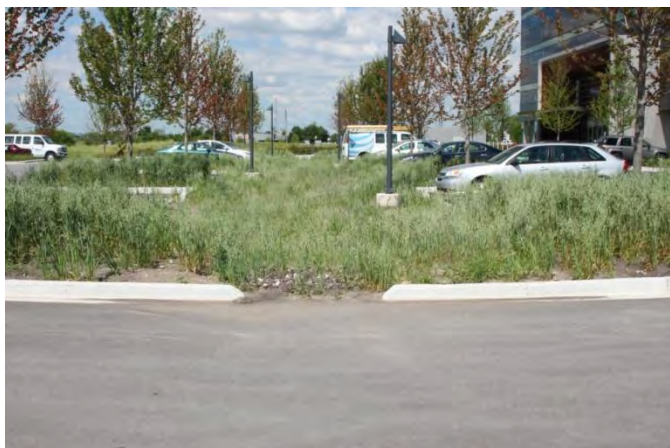
Figure 3-3. Bioretention, Panduit Building, Tinley Park
