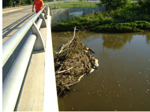
Figure 3-5. Woody Debris Accumulation, Hickory Creek at Cedar Road, New Lenox
