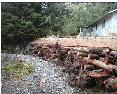
Figure 4-39. Log Cribbing, Salmon Creek, WA (Source: Inter-Fluve, Inc.)
