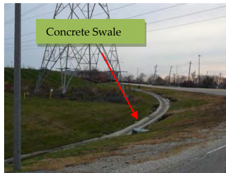
Figure 4-20. Concrete-Lined Ditch, Degroate Road, New Lenox
