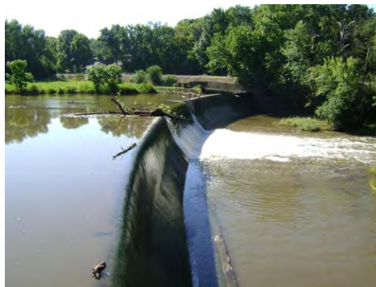
Figure 4-36. Pilcher Park Dam, Joliet
