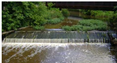
Figure 4-35. Spring Creek Dam at Draper Avenue, Joliet
