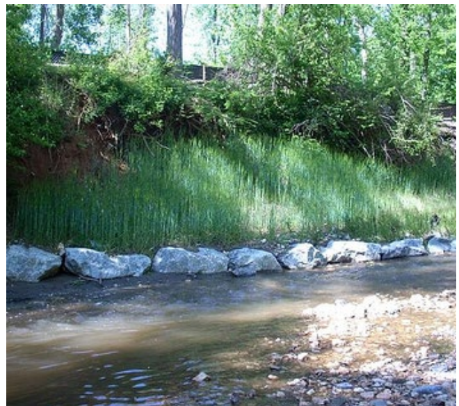
Stone toe protection, which prevents streambank erosion and shoreline erosion. Photo: Montgomery County, Maryland.
