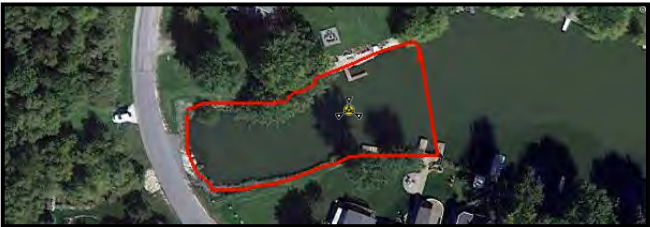
Photo of the Northwest Basin
