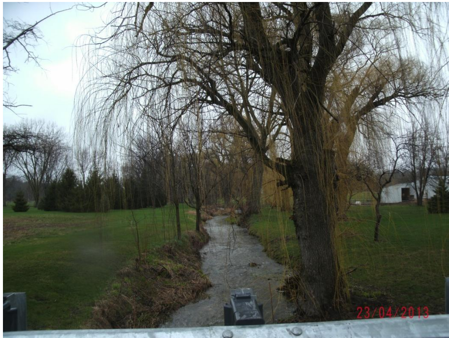
Spring Brook Looking Upstream of Orth Rd.
