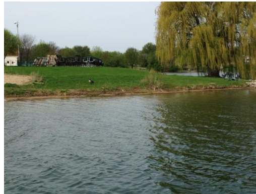
An eroding shoreline at Candlewick Lake (left).
