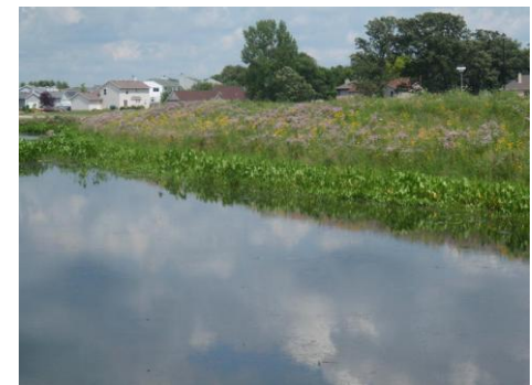
Constructed wetlands around a basin were created by Olson Ecological Solutions (Hoffman).
