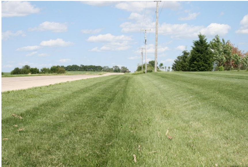
Figure 16: Grassed swale along a roadside.
