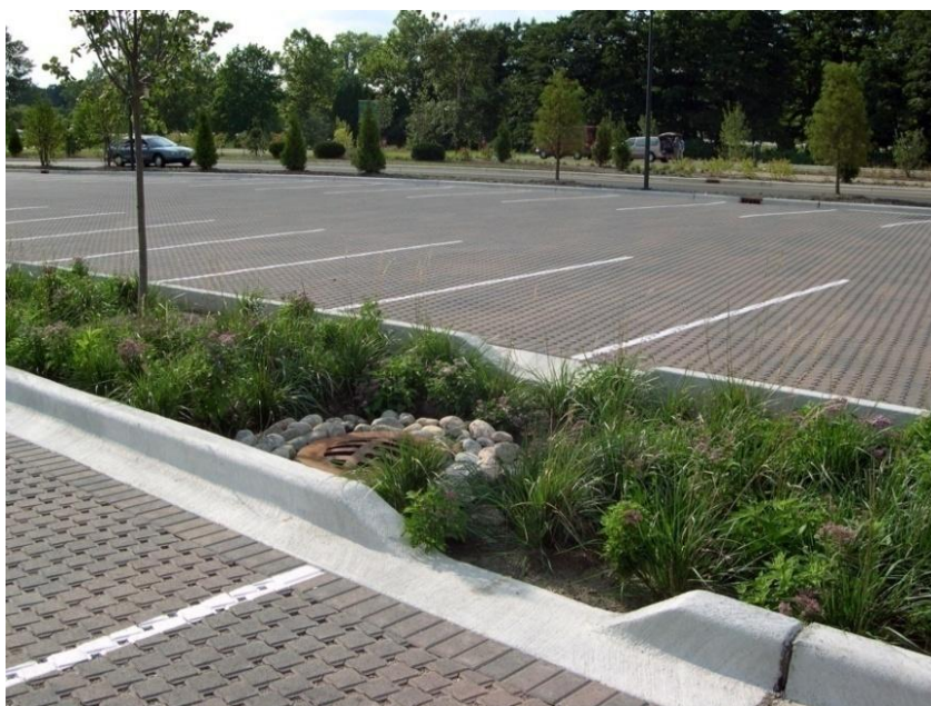
Figure 18: Permeable paver parking lot with bioswales.
