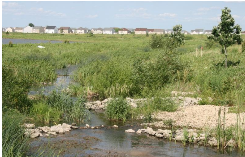
Figure 21: Stabilized stream channel adjacent to a stormwater basin in Joliet, IL
