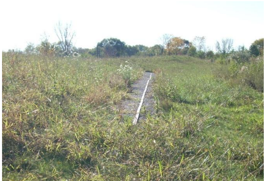
Figure 20: Level spreader outlet used in a recently restored riparian buffer.
