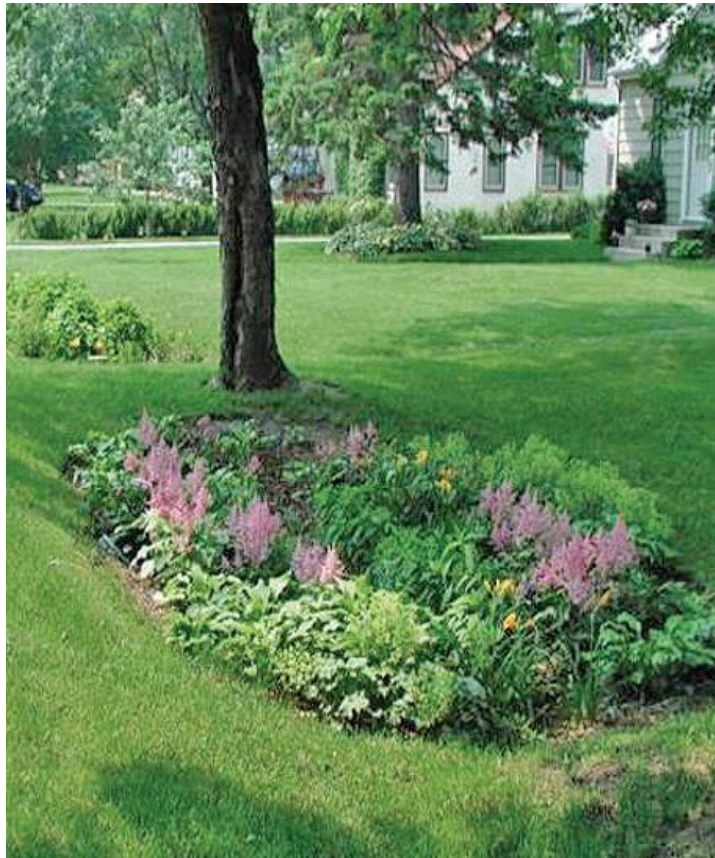
Figure 17: A rain garden created at the base of an embankment of a roadway.
