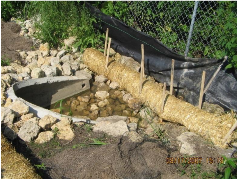
Figure 23: Coir logs installed at a stormwater outlet (flared end section at the end of the treatment train) along with rip-rap to prevent sediment from leaving the site at the edge of the property.
