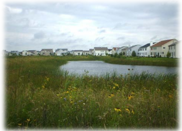
Naturalized Detention Basin
