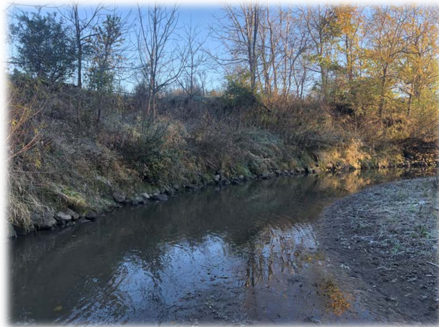
Existing Streambank Stabilization
