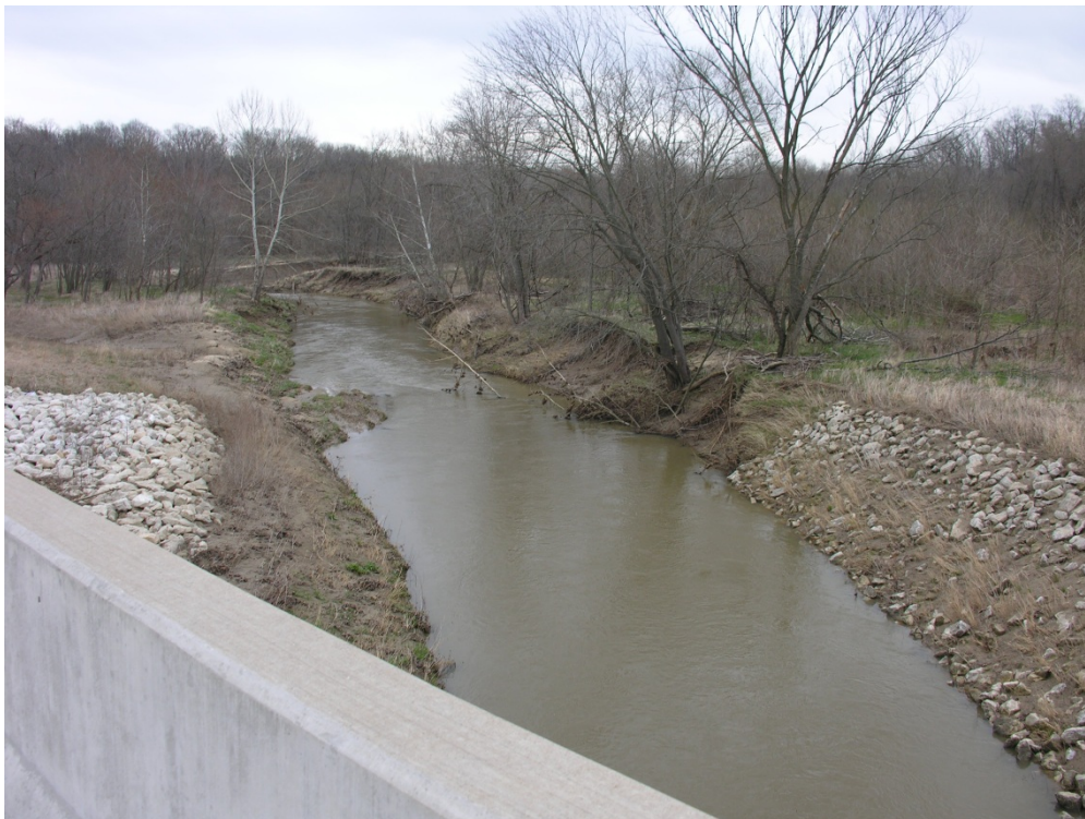
Figure 2-1. Sugar Creek at U.S. Route 24, looking downstream
