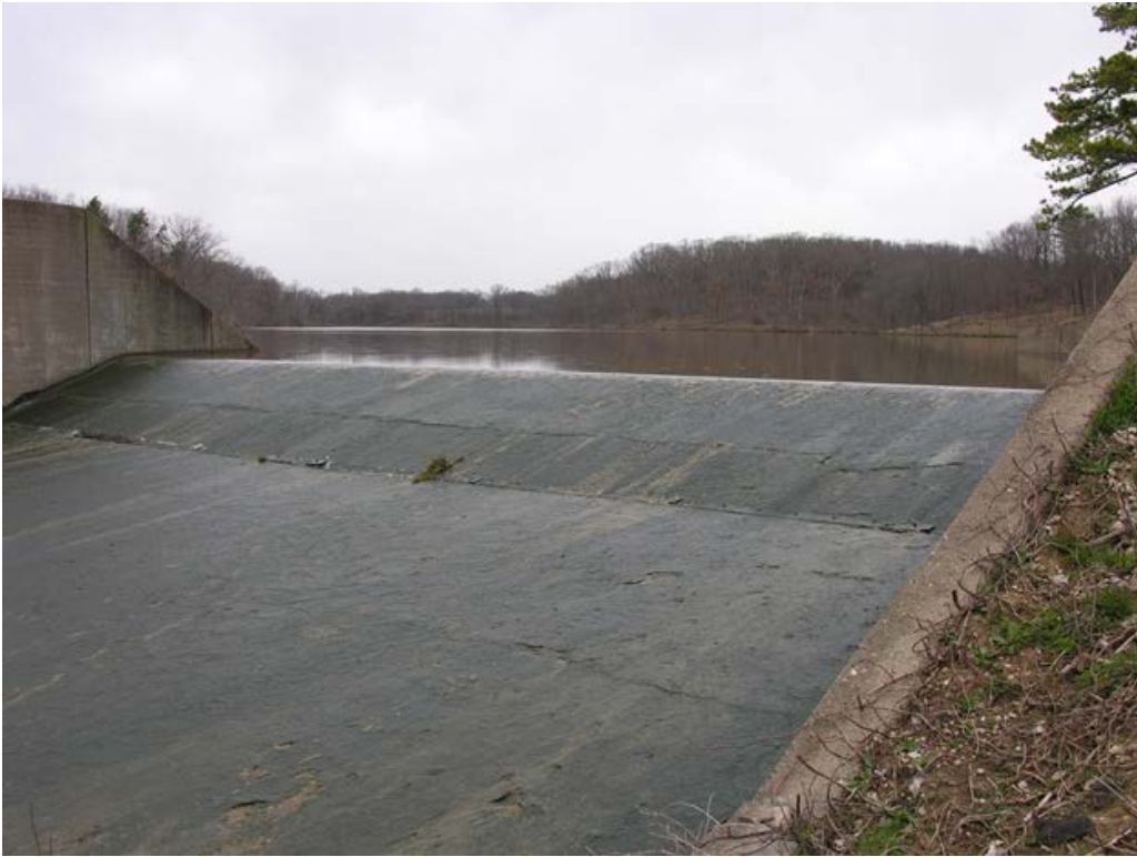
Figure 5-3. Vermont City Reservoir spillway
