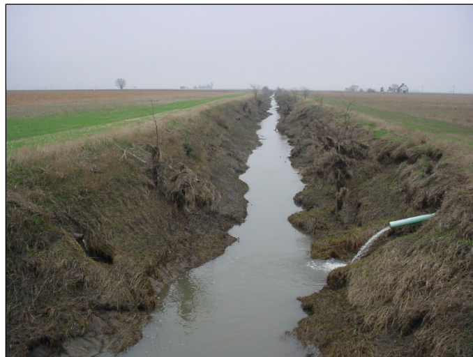
Figure 7. Drain tile discharging into the North Fork Vermilion Tributary.
