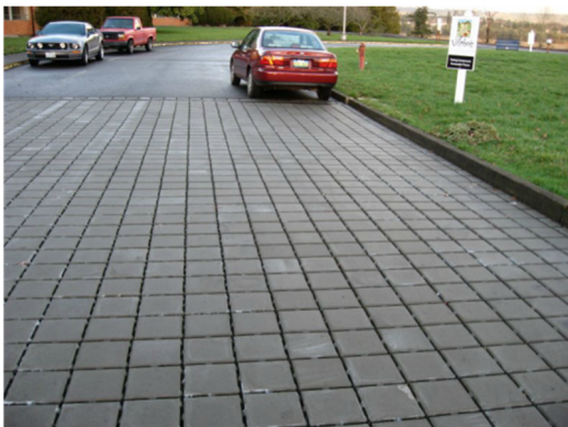
Permeable pavement (NCSWCD 2017)
