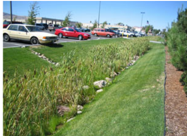
Vegetated swales (Dott Architecture 2010)
