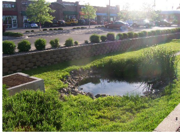
Stormwater retention basin (USEPA 2016a)
