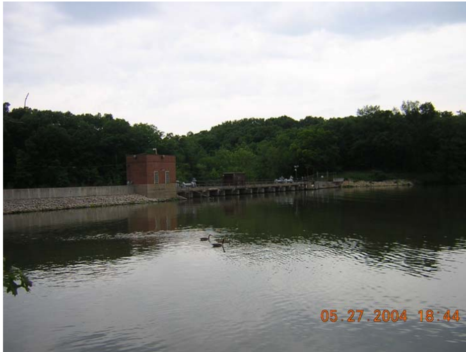
Lake Vermilion Dam and Spillway
