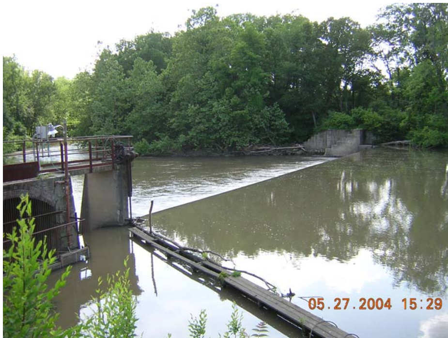
Water Plant Intake
