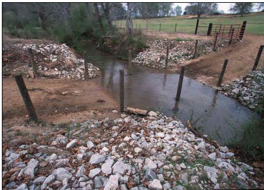
Figure 4-12. Restricted Cattle Access Point with Reinforced Banks.
