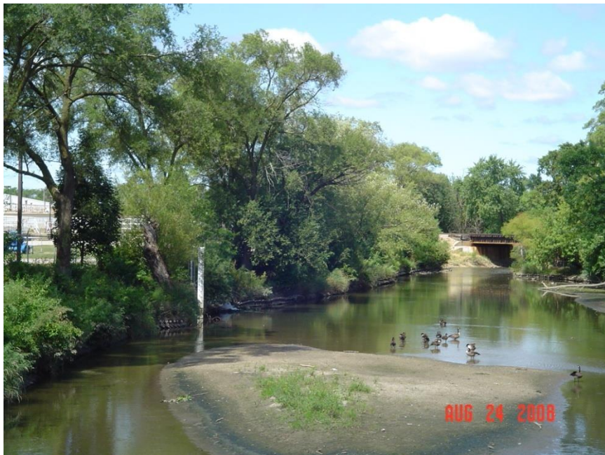
Salt Creek (IL_GL-10) at Route 19
