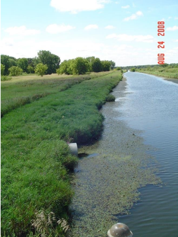
Salt Creek (IL_GL) at Route 58
