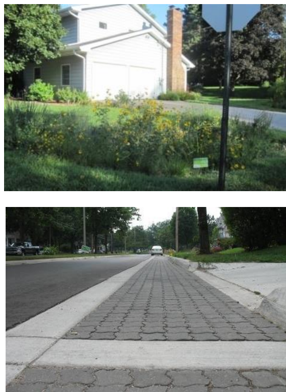
Figure 76. Green infrastructure examples: top - residential rain garden; bottom - permeable pavement.
