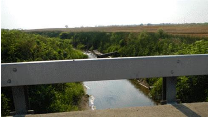
Unnamed tributary to Bonpas Creek at 270 East
