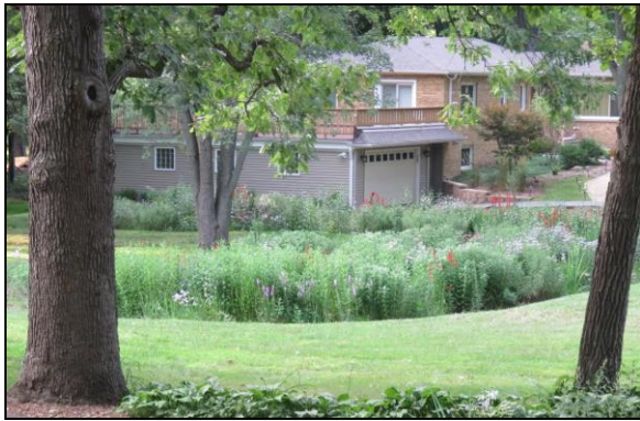
Bioswale post-construction.
