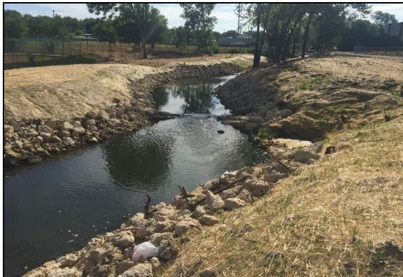
Streambank stabilization post-construction.
