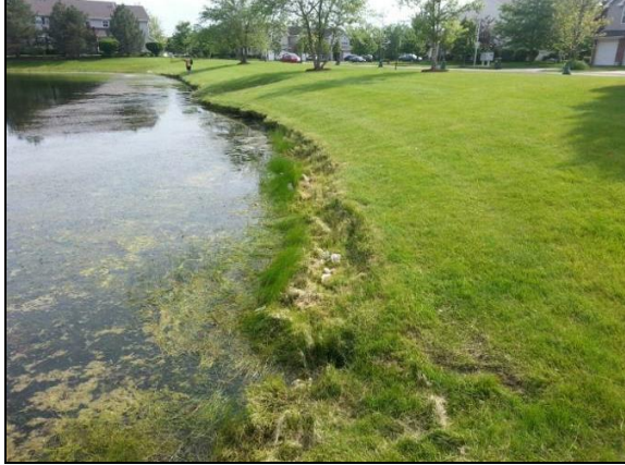
Shoreline stabilization pre-construction.
