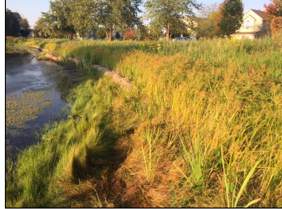
Shoreline stabilization post-construction.
