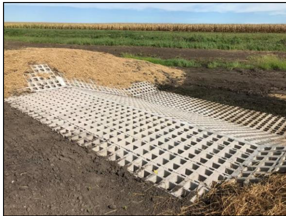
Block chute post-construction.
