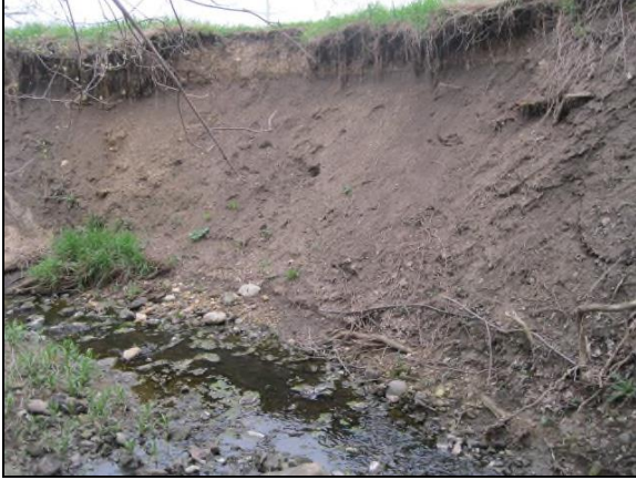
Streambank stabilization pre-construction.
