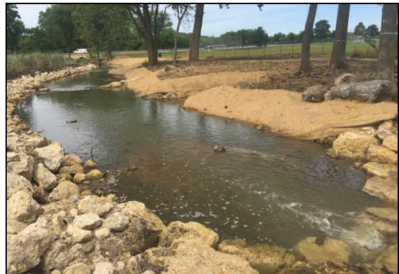
Streambank stabilization post-construction.
