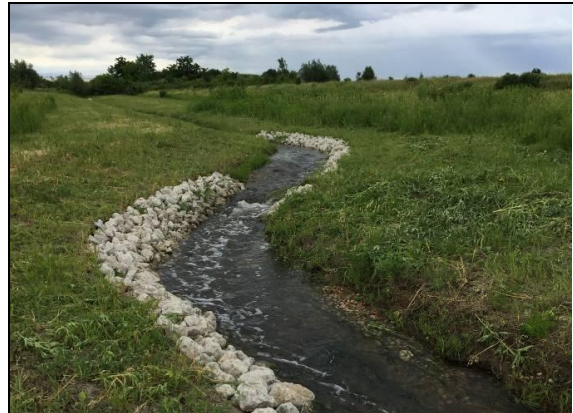
Woods Creek bank stabilization post-construction.
