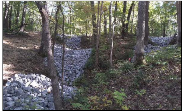
Gully stabilization post-construction.
