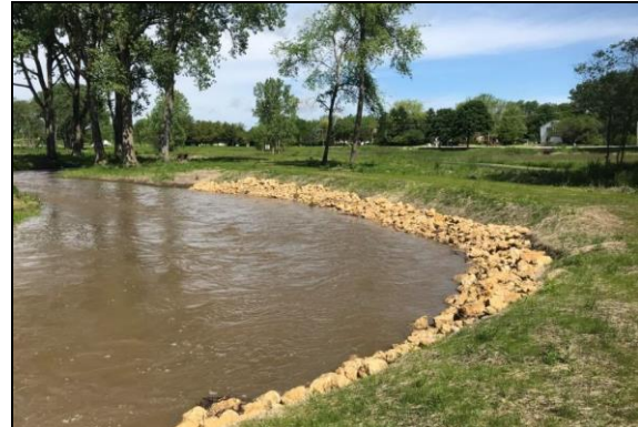
Streambank stabilization post-construction.
