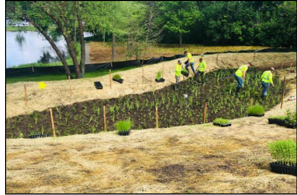
Stormwater wetland during construction.
