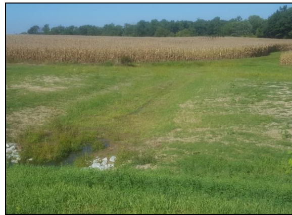
Grassed waterway post-construction.
