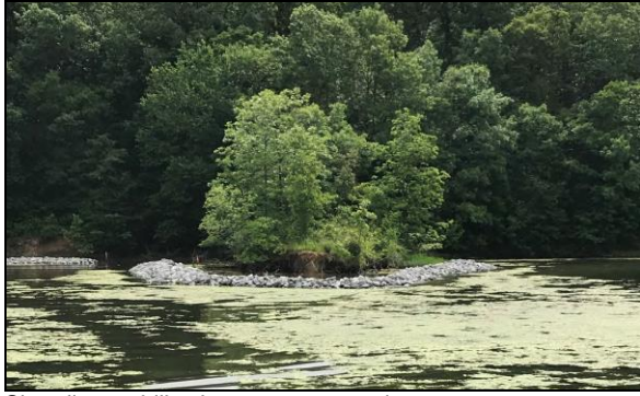
Shoreline stabilization post-construction.
