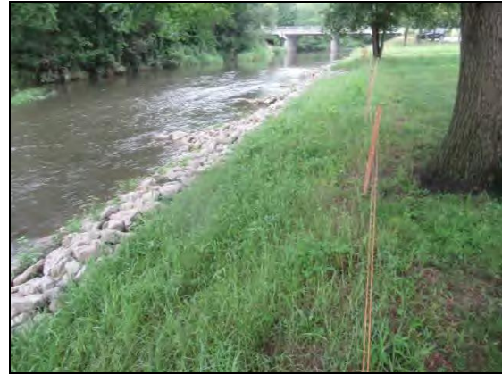
Hickory Creek bank stabilization post-construction.
