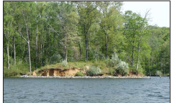
Kinkaid Lake shoreline stabilization post-construction.
