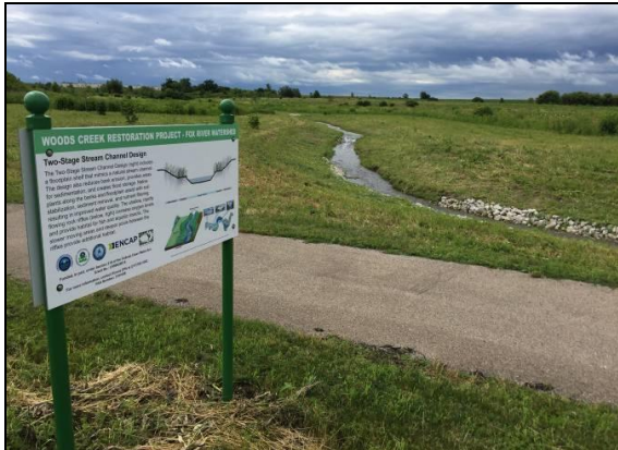
Woods Creek bank stabilization post-construction.
