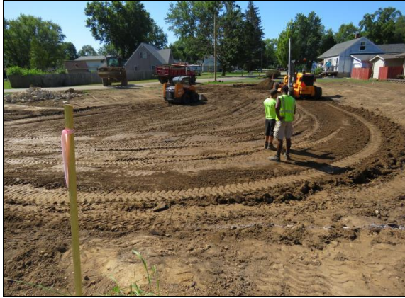
West bioretention basin during construction.
