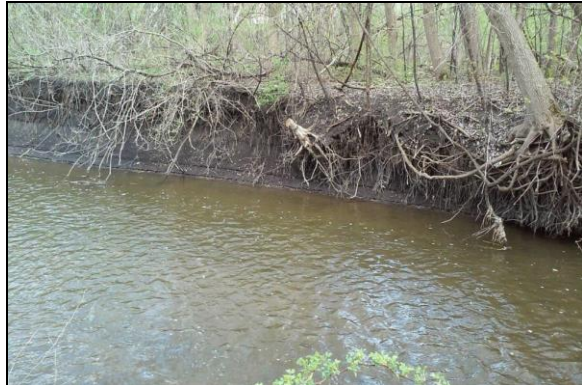
Streambank stabilization pre-construction.
