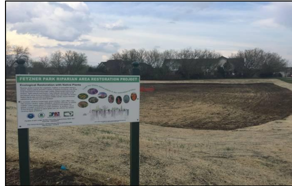
Detention basin retrofit post-construction.
