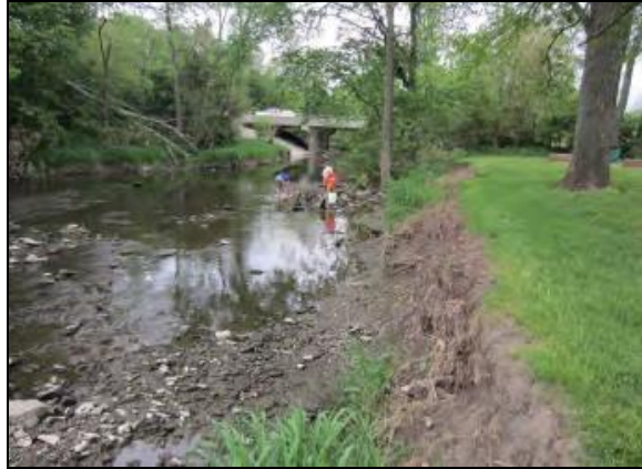
Hickory Creek bank stabilization pre-construction.
