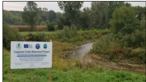
Streambank stabilization post-construction.
