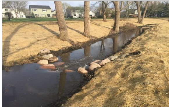
Streambank stabilization post-construction.
