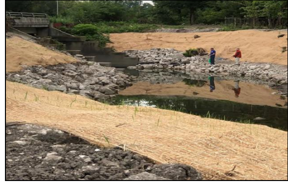
Streambank stabilization post-construction.
