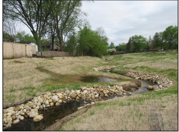
Streambank stabilization post-construction.
