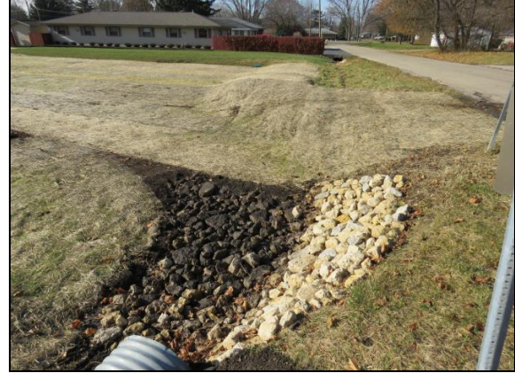
West bioretention basin post-construction.
