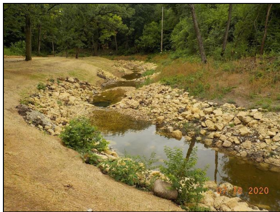
Streambank stabilization post-construction.
