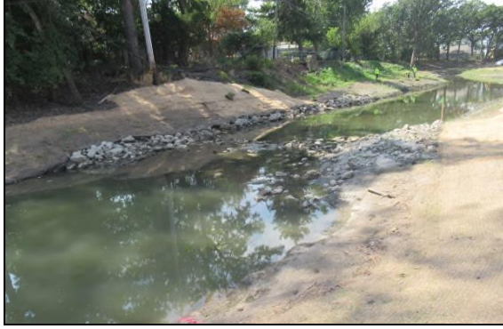
Streambank stabilization post-construction.
