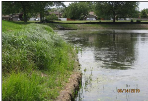
Shoreline buffer filter strip post-construction.
