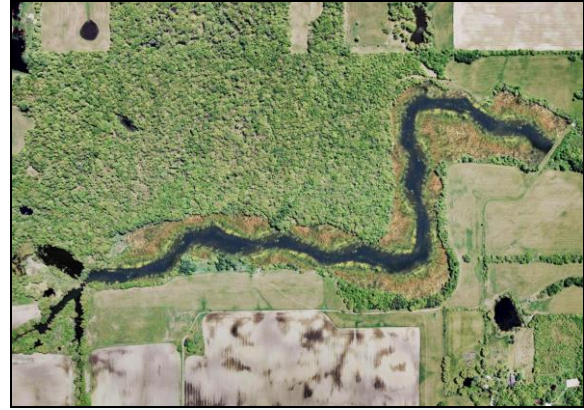
North Mill Creek restoration post-construction.
