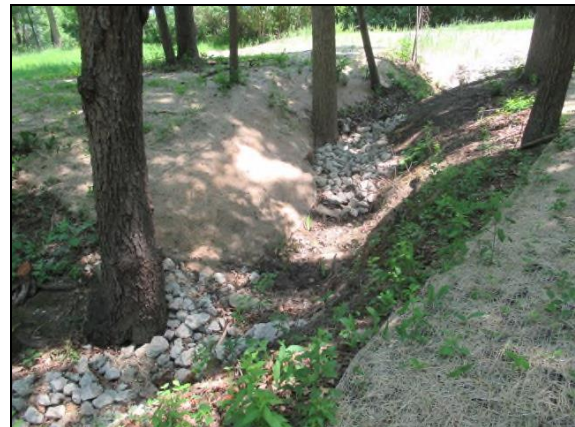
Stream channel stabilization post-construction.
