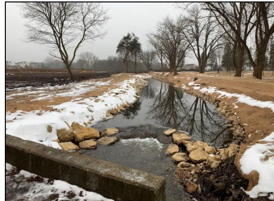
Streambank stabilization post-construction.
