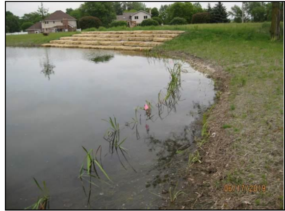
Urban stormwater wetland post-construction.
