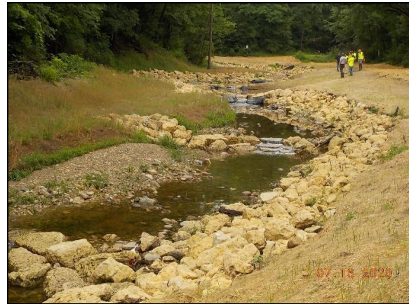
Streambank stabilization post-construction.
