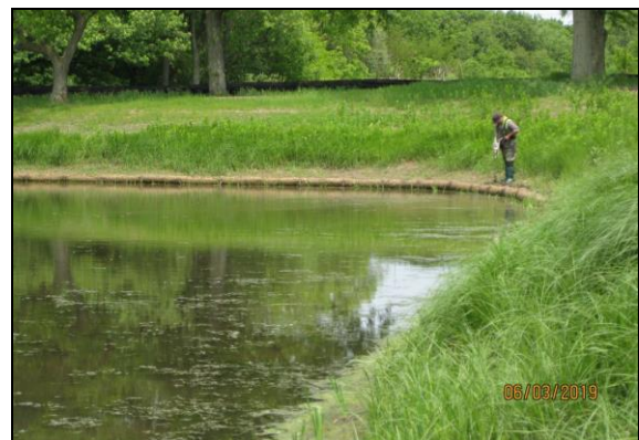
Shoreline buffer filter strip post-construction.
