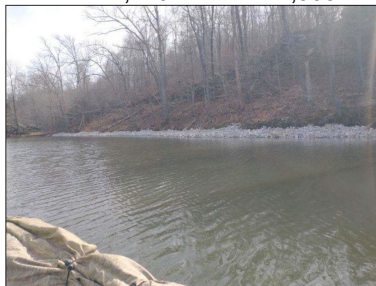
Finished Product of Bank Stabilization
