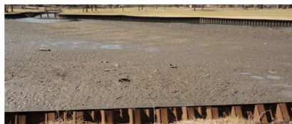
Photo 6: Pre-construction shallow water depths at the impounded area result in exposure of mud flats with a water level of drawdown of 0.75 feet. The completed project used these conditions to construct wetland, a sediment forebay, a restored stream channel, and other water quality improvements.
