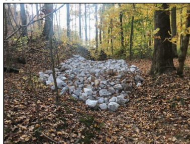
Finished Product of Gully Stabilization
