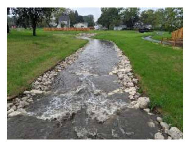
FAA 3191810 – The 7<sup>th</sup> Avenue Creek Stream Restoration Project stabilized eroding streambanks along the 7<sup>th</sup> Avenue Creek in St. Charles, Illinois.
