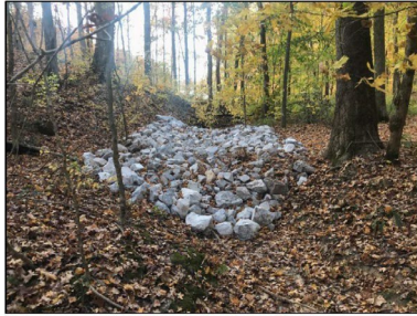
Finished Product of Gully Stabilization
