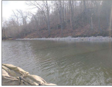
Finished Product of Bank Stabilization
