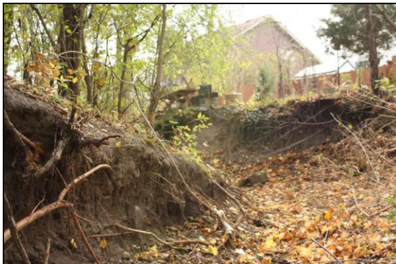
Carpenter Creek pre-construction.
