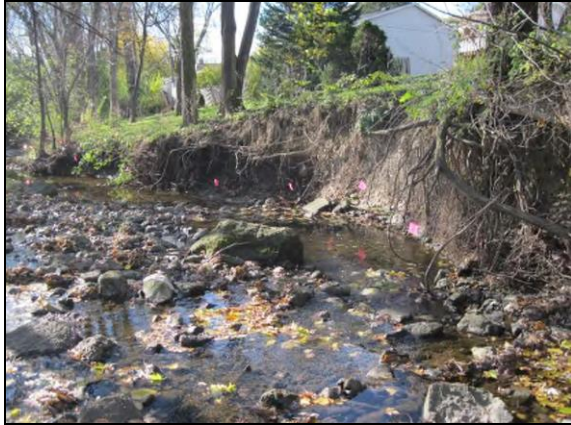
Crabtree Creek bank stabilization pre-construction.
