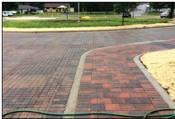
Edgewood School permeable pavement post-construction.
