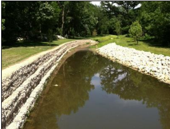
Babbling Brook bank stabilization post-construction.
