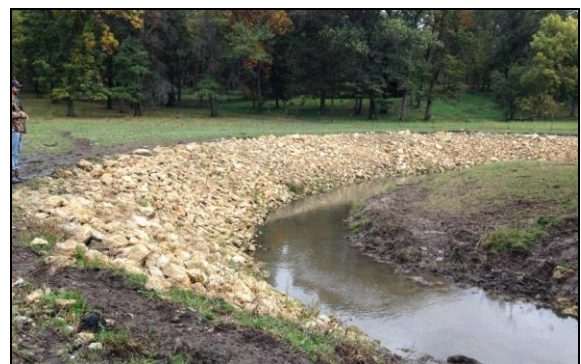
Babbling Brook restoration post-construction.
