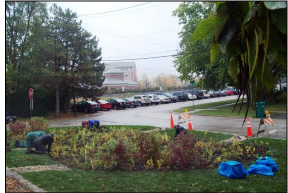
Metra parking lot rain garden post-construction.
