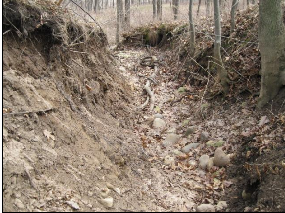
Silver Creek tributary stabilization pre-construction.
