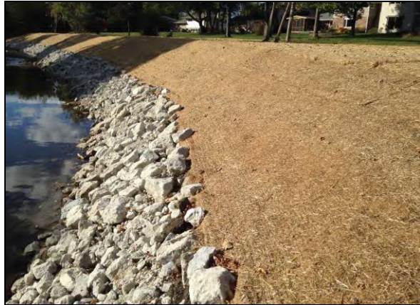
Salt Creek bank stabilization post-construction.
