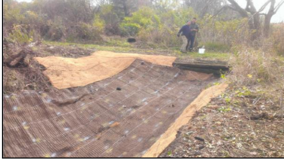
Ditch (gully) stabilization during construction.
