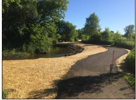
Otter Creek stabilization post-construction.
