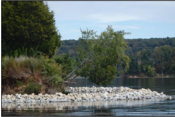
Cedar Lake shoreline stabilization post-construction.
