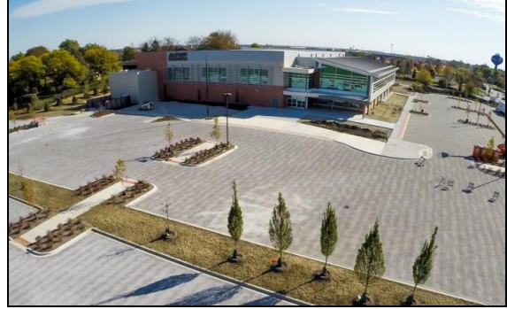
Permeable pavement parking lot post-construction.
