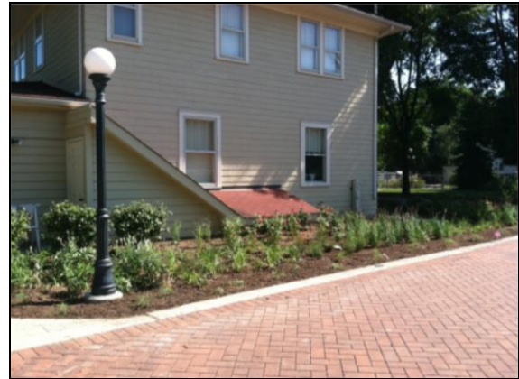
Rain garden and permeable pavement post-construction.
