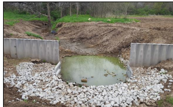
Aluminum toewall grade stabilization post-construction.
