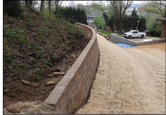
Grade stabilization structure post-construction.
