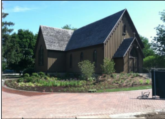
Rain garden and permeable pavement post-construction.
