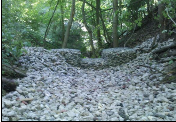
Grade stabilization structure post-construction.
