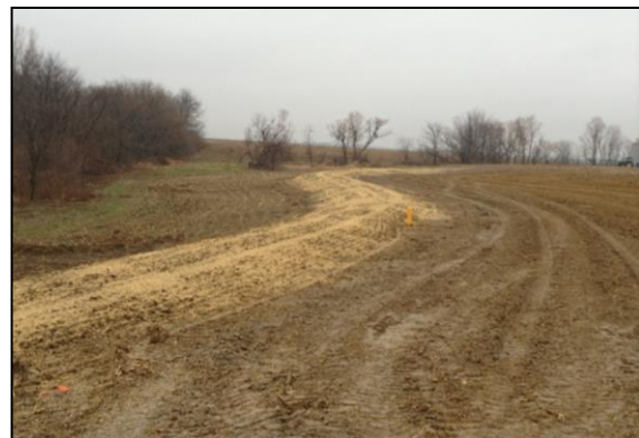
Water & sediment control basin / terrace post-construction.
