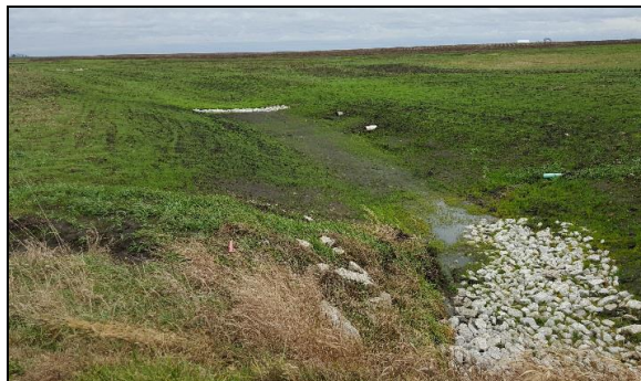
Grassed waterway with rock checks post-construction.
