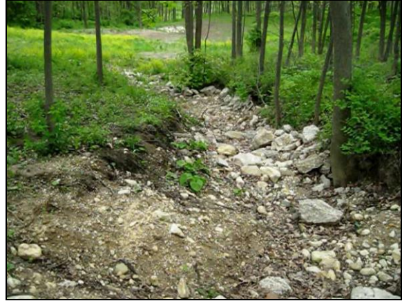
Silver Creek tributary stabilization post-construction.
