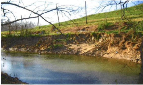
Stream channel restoration pre-construction.
