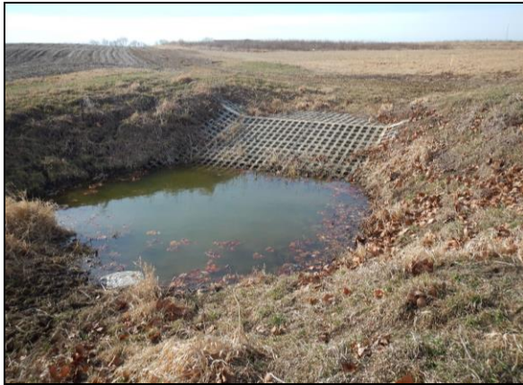
Block chute grade stabilization post-construction.
