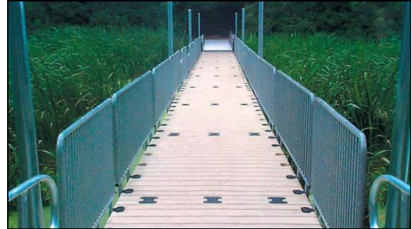
Elevated boardwalk over wetland post-construction.
