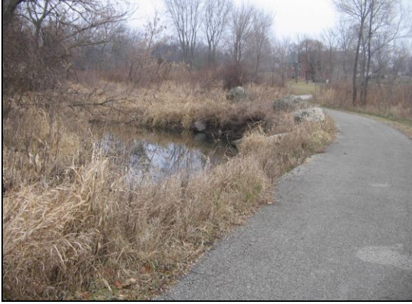
Otter Creek stabilization pre-construction.
