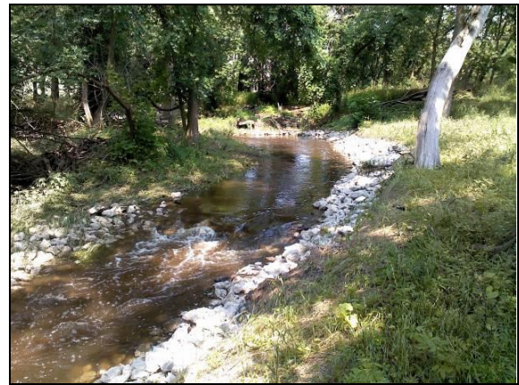
North Flint Creek stabilization post-construction.
