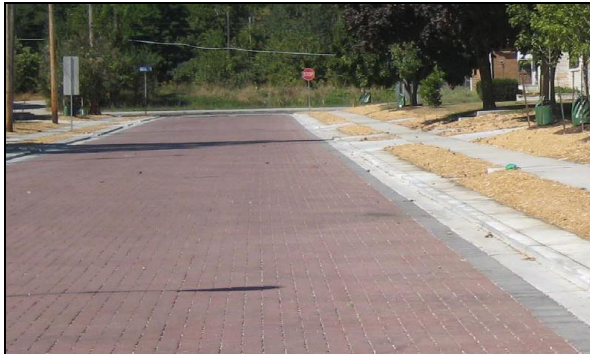
Permeable pavement post-construction.
