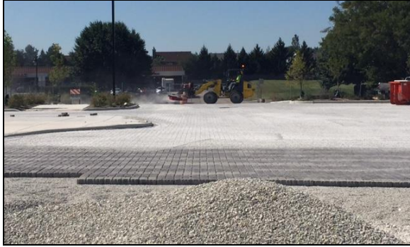
Permeable pavement parking lot during construction.
