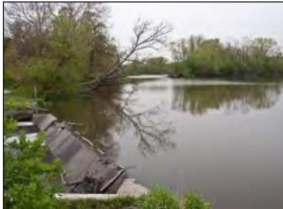
Dam modification pre-construction.
