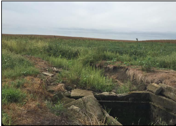
Grassed waterway pre-construction.
