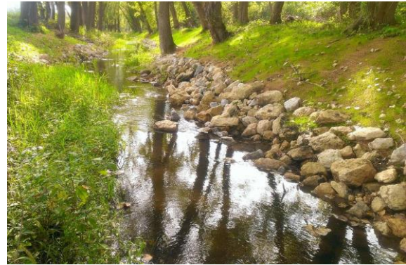
Galt Creek bank stabilization post-construction.
