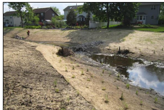
Carpenter Creek stabilization post-construction.
