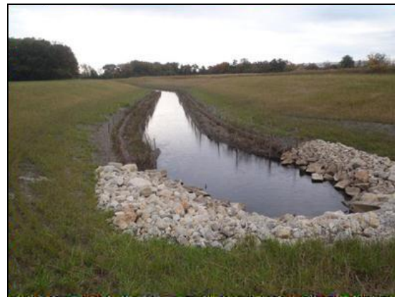
Skokie River daylighting post-construction.
