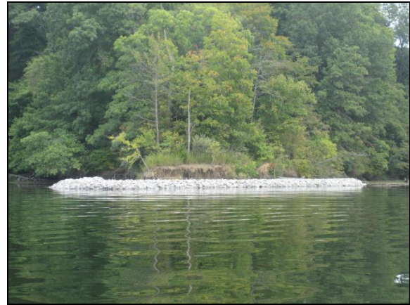
Kinkaid Lake off-shore breakwater post-construction.
