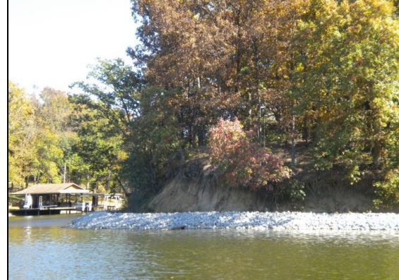
Lake Sara shoreline stabilization post-construction.
