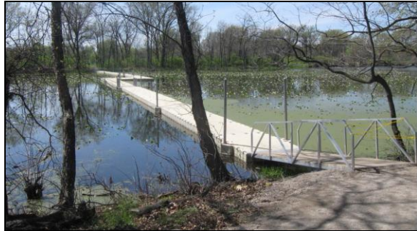
Elevated boardwalk over wetland during construction.
