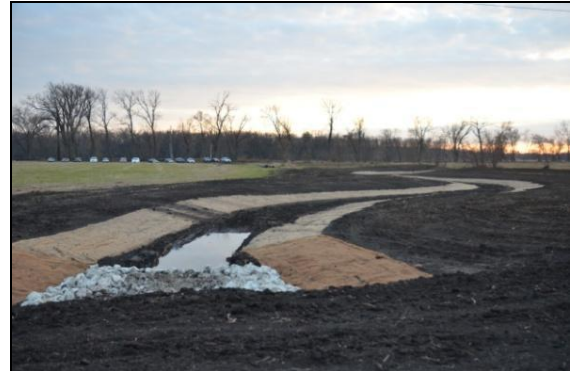
Stream channel restoration post-construction.
