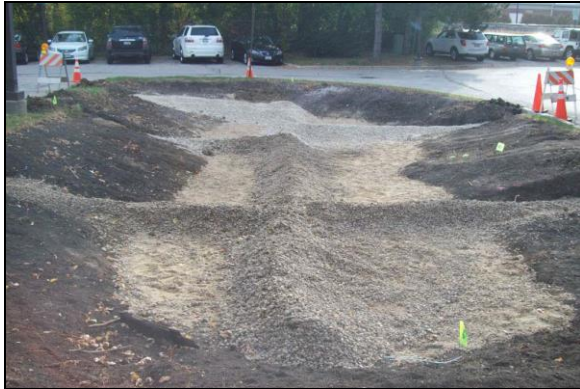
Metra parking lot rain garden during construction.
