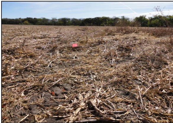
Water and sediment control basin pre-construction.
