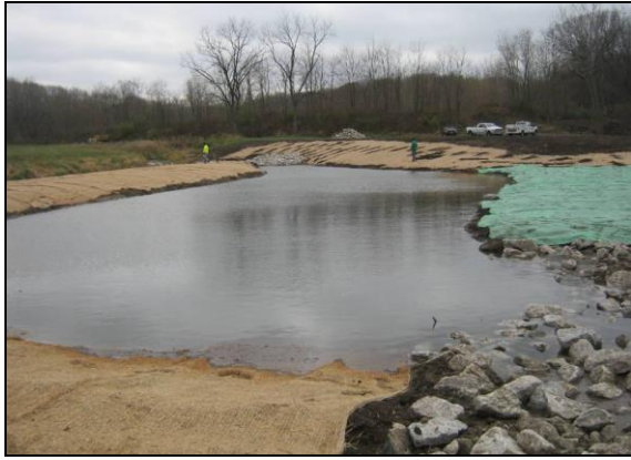
Basin during construction.
