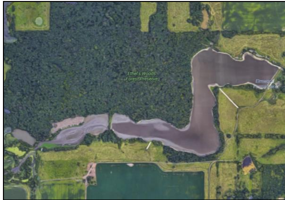
North Mill Creek restoration pre-construction.
