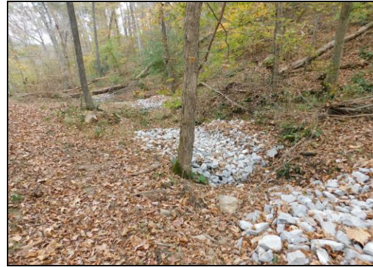
Gully stabilization post-construction.
