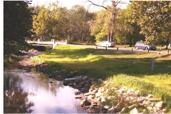
Tyler Creek bank stabilization post-construction.
