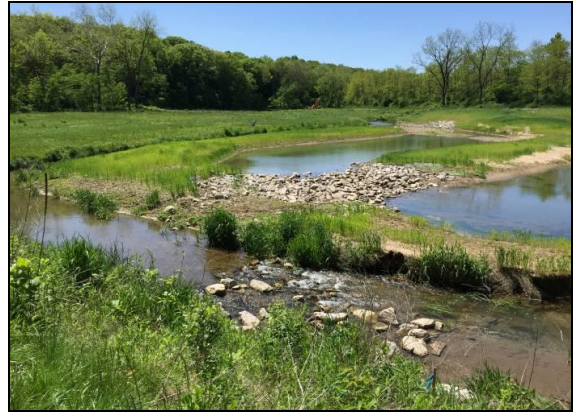
Riffle and weir connecting the two basins post-construction.
