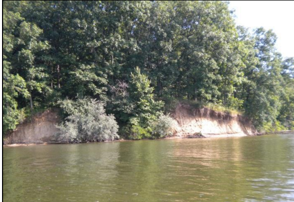
Lake Sara shoreline stabilization pre-construction.
