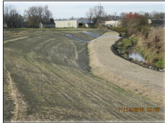
Two-stage ditch post-construction.
