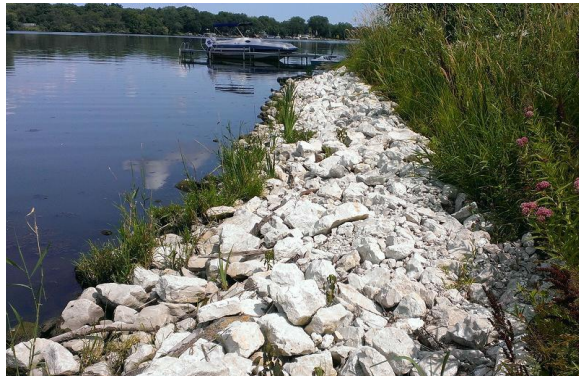
Wonder Lake shoreline stabilization post-construction.
