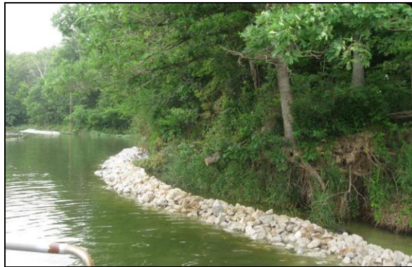
Otter Lake shoreline stabilization post-construction.
