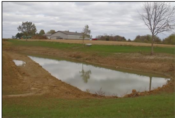
Sediment basin post-construction.
