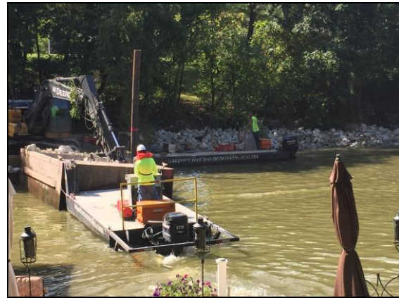
Shoreline stabilization during construction.
