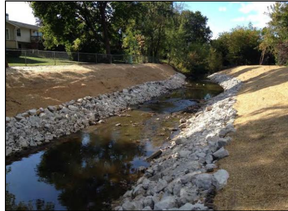
Salt Creek bank stabilization post-construction.
