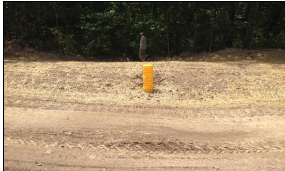
Water and sediment control basin post construction.
