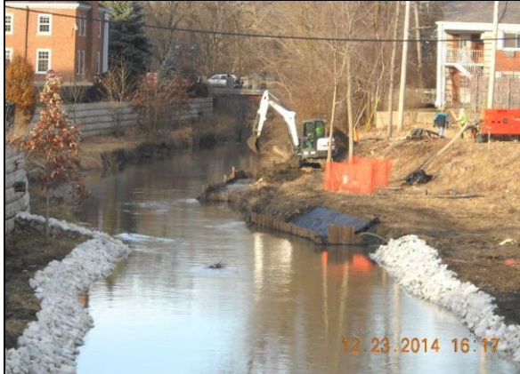
W. Fk. N. Br. Chicago River stabilization during-construction.
