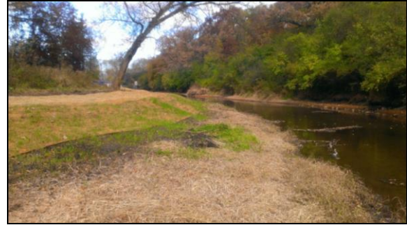
Nippersink Creek bank stabilization post-construction.
