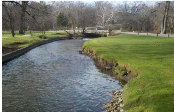
Tyler Creek bank stabilization pre-construction.
