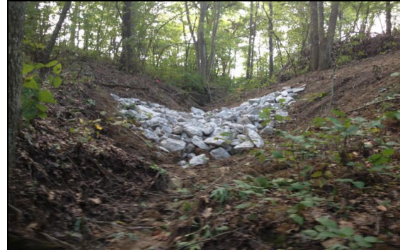
Grade stabilization structure post-construction.
