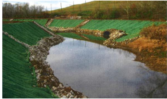
Stream channel restoration post-construction.
