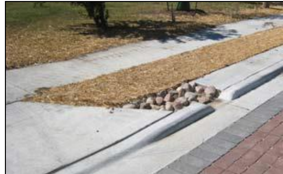
Cobble curb cuts and infiltration channel post-construction.
