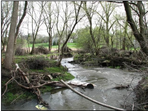
North Flint Creek stabilization pre-construction.
