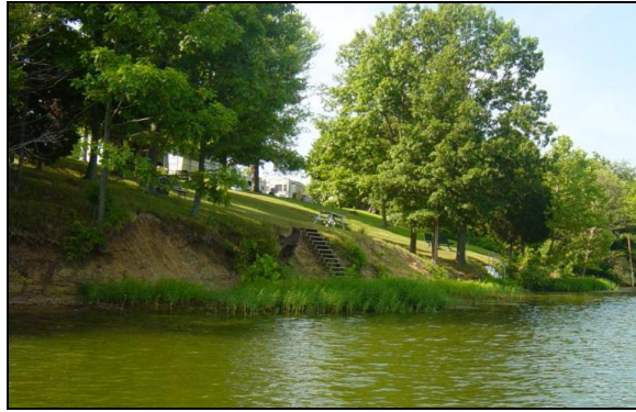
Kinkaid Lake shoreline stabilization pre-construction.
