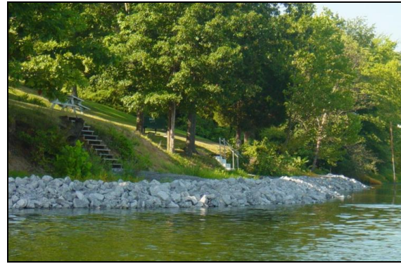
Kinkaid Lake shoreline stabilization post-construction
