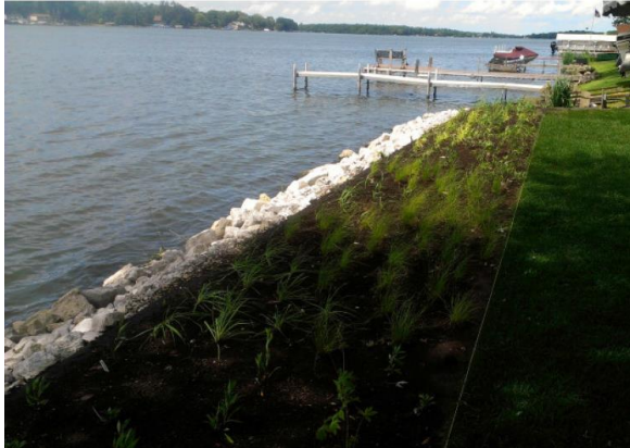
Wonder Lake shoreline stabilization post-construction.
