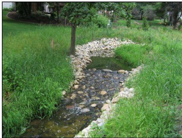
Hobson Creek stabilization post-construction.
