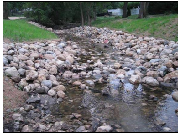
Crabtree Creek bank stabilization post-construction.
