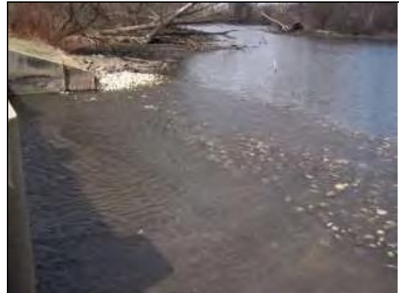
Dam modification post-construction.
