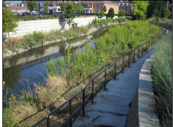
W. Fk. N. Br. Chicago River stabilization post-construction.
