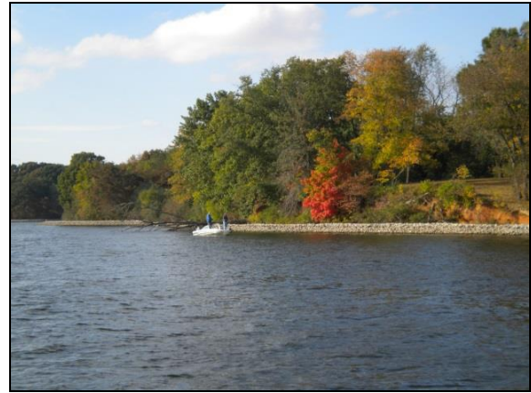
Lake Sara shoreline stabilization post-construction.
