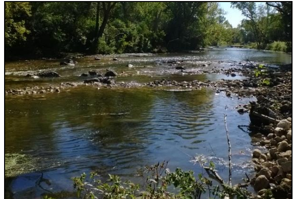
W. Br. DuPage River channel stabilization post-construction.
