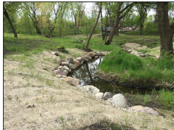
Bull Creek bank stabilization post-construction.
