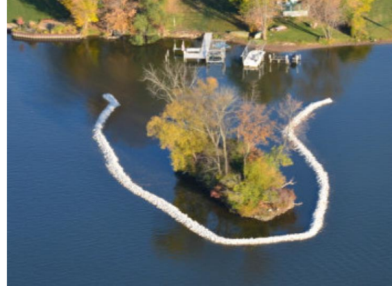
Wonder Lake shoreline stabilization post-construction.
