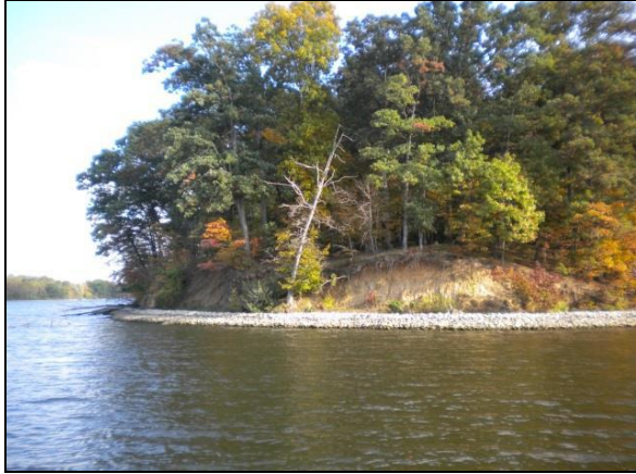
Lake Sara shoreline stabilization post-construction.
