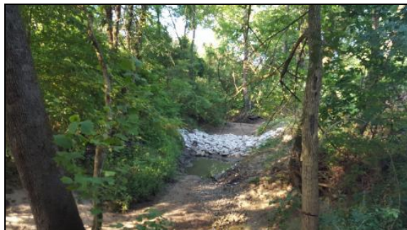
Stream channel stabilization post-construction.
