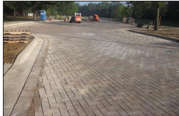
Seager Park permeable pavement during construction.
