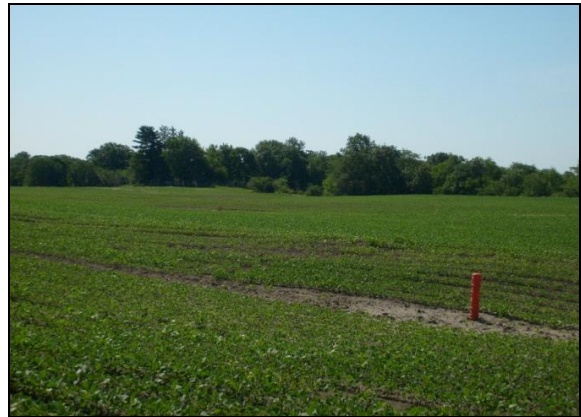
Water and sediment control basin post-construction.
