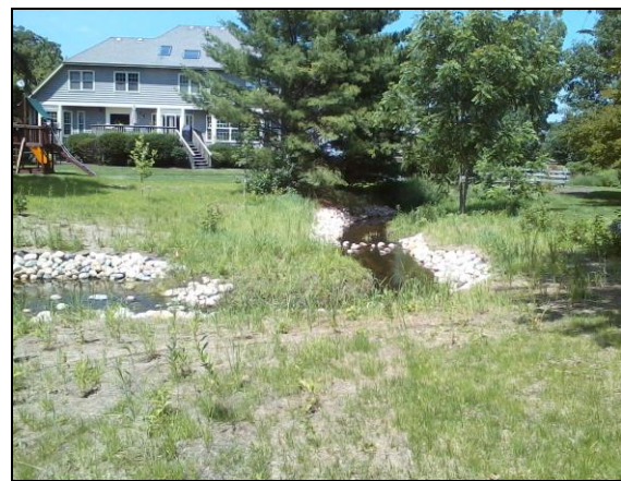
Hobson Creek stabilization post-construction.
