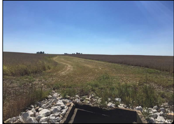
Grassed waterway post-construction.
