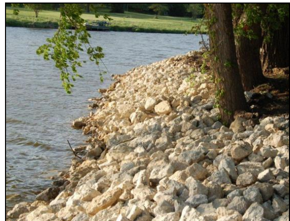
Lost Nation Lake shoreline stabilization post-construction.
