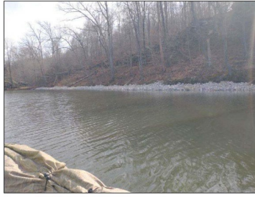
Finished Product of Bank Stabilization
