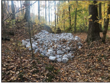
Finished Product of Gully Stabilization
