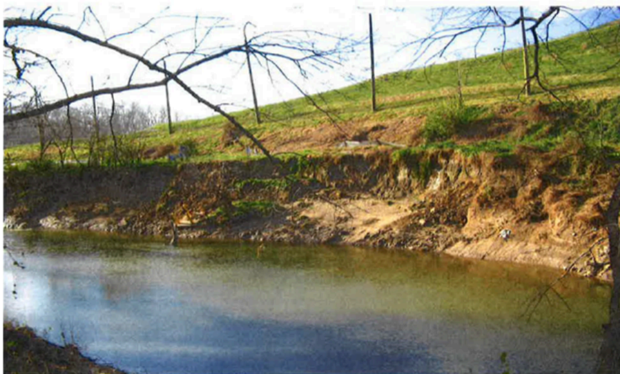
Figure 1. Typical bank erosion before project
