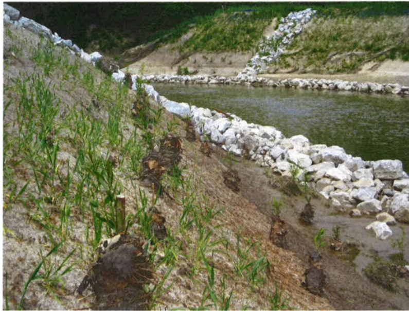
Willow stakes planted March 2014 growing on streambank May 22, 2014. Notice leaves and debris around willow stakes left by spring floods.
