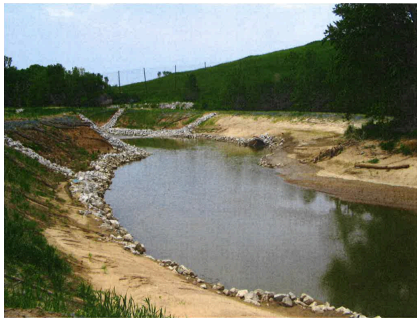
Looking downstream at lower Rock Riffle structure and Fish Passage Structure on May 22, 2014
