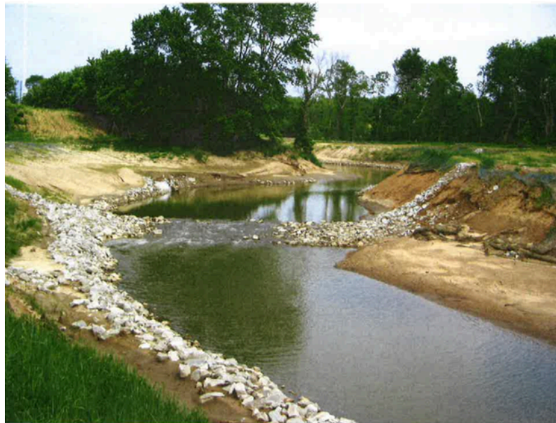
Looking upstream at upper Rock Riffle structure and Fish Passage structure spring 2014
