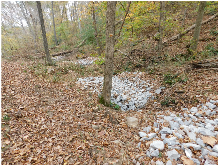
Figure 3. Finished gully stabilization from the 2015 project.
