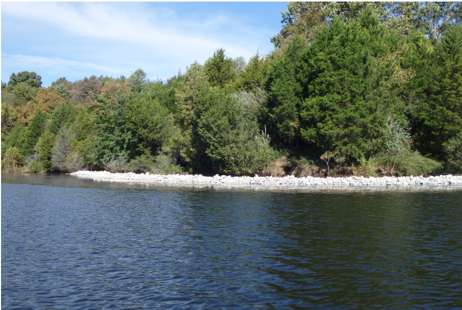
Figure 2. Finished section of shoreline stabilization from the 2015 project.
