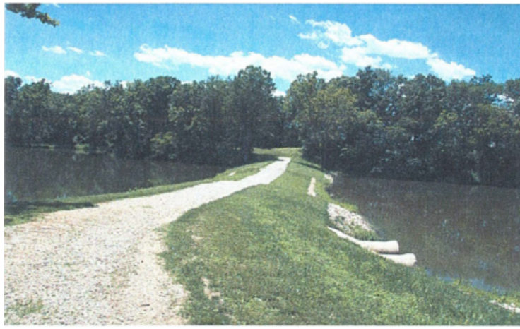
Figure 3. Completed control structure
