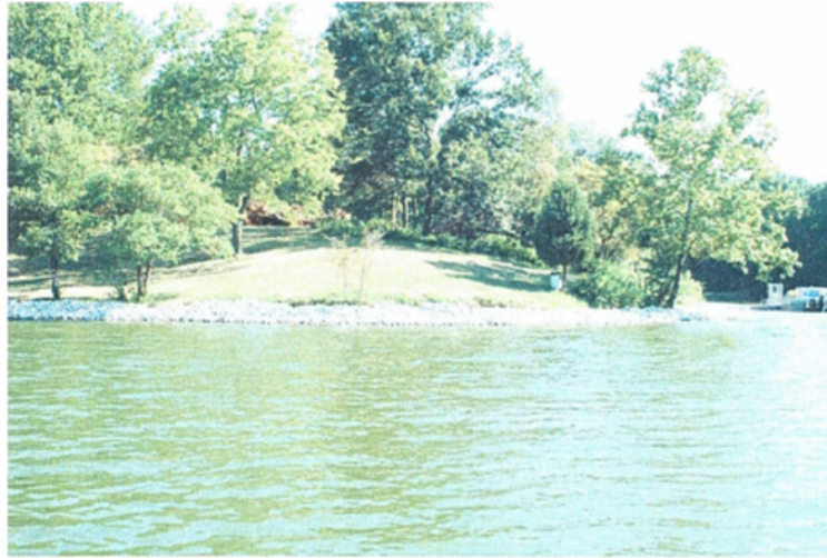
Figure 2. Riprap revetment
