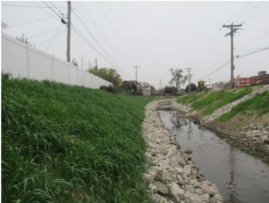
Figure 5. Post-construction photograph of streambank stabilization for Silver Creek after vegetation has begun to establish
