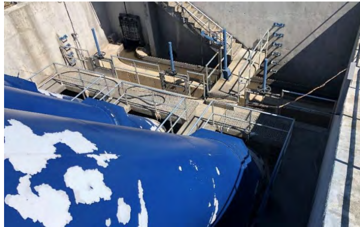
Figure 5-5 Stormwater Diversion Structure
