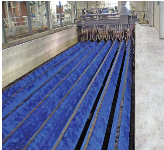
Figure 6-4 Diamond Filter Cloth Laterals
