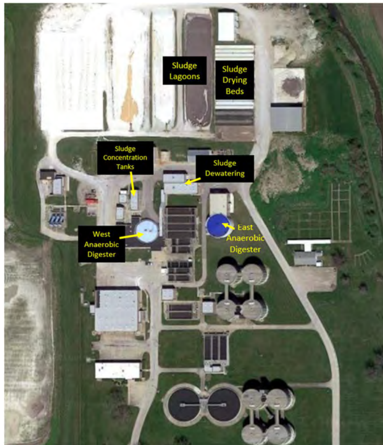
Figure 5-13 Locations of Solids Handling Units
