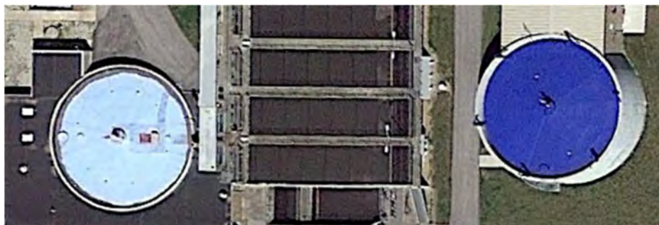
Figure 5-14 West Anaerobic Digester (left) and East Anaerobic Digester (right)
