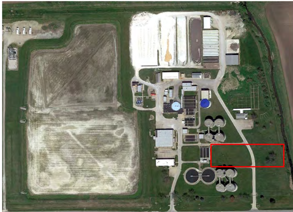
Figure 3-2 Wastewater Treatment Plant Aerial Photo
