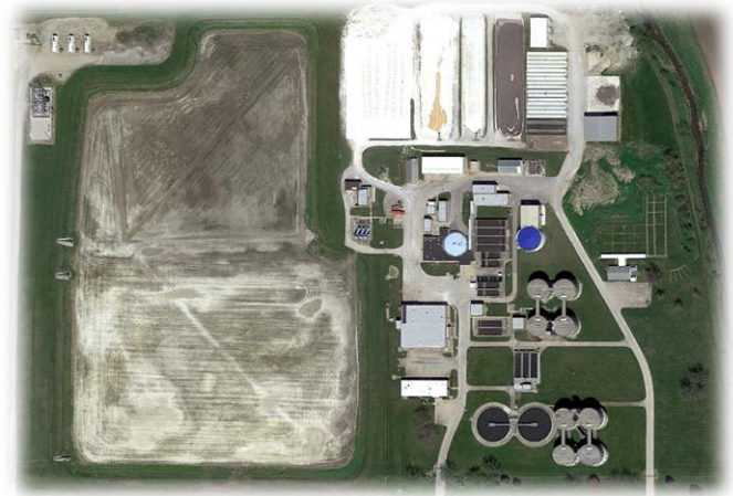
Village of Rantoul WWTP
