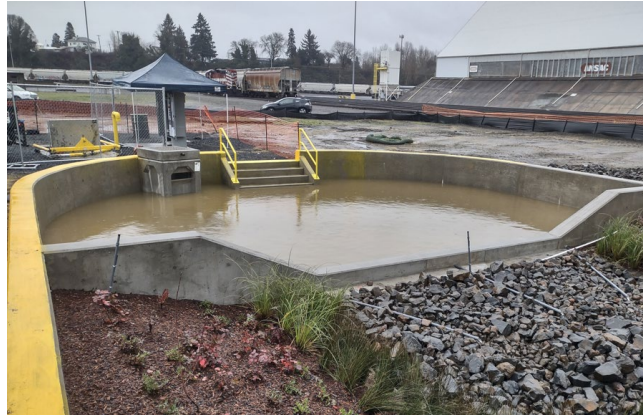
Example of Pretreatment device: Sedimentation Forebay
