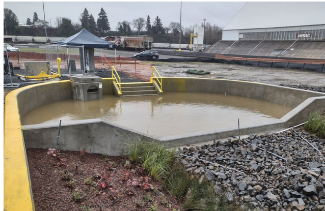
Example of Pretreatment device: Sedimentation Forebay
