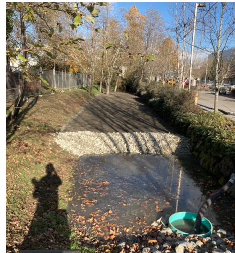
Example of a Filtration Basin with Engineered Media for Phosphorus Removal
