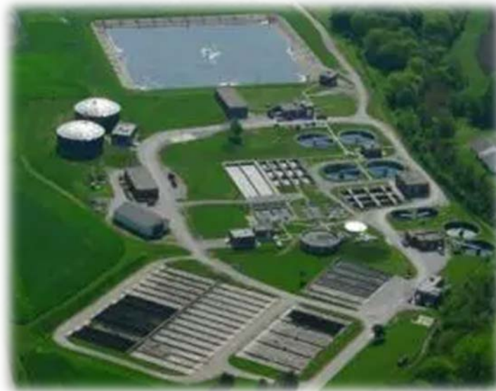
City of Mattoon Treatment Plant
