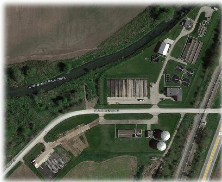
Aqua Illinois Manteno Treatment Plant
