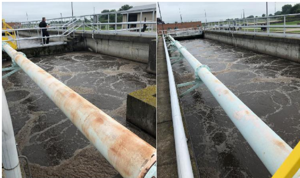
Figure 3-6: West Aeration Basin
