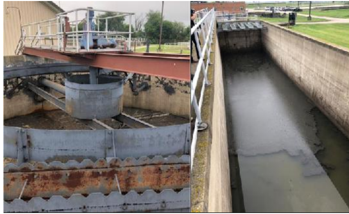
Figure 3-11: Circular (left) and Rectangular (right) Excess Flow Clarifiers
