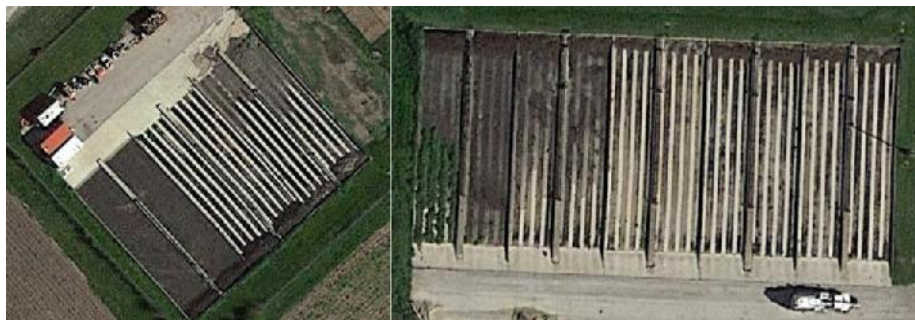
Figure 3-16: Southwest (left) and North (right) Sludge Drying Beds
