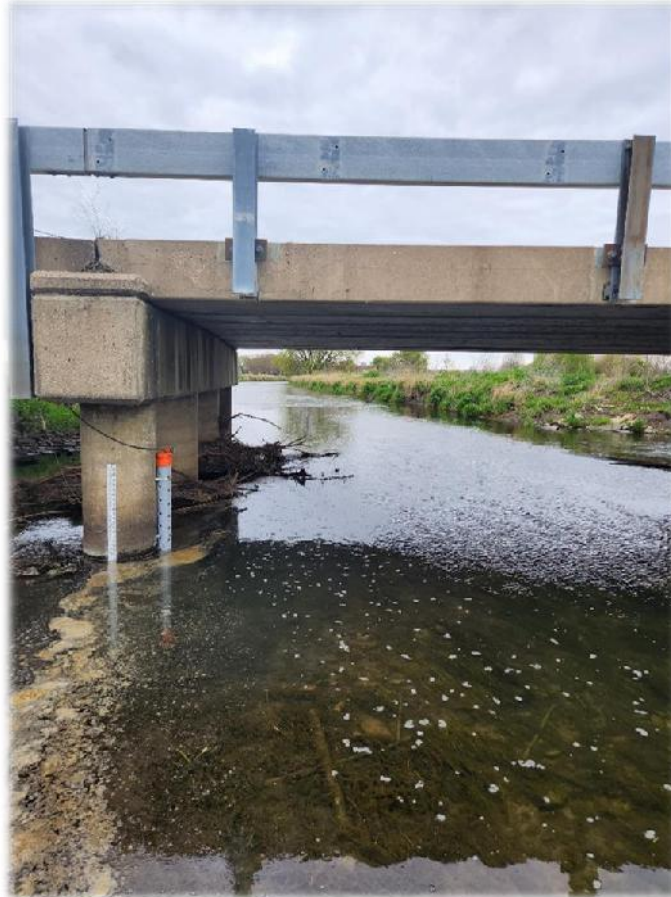
Example of infrastructure at South Branch Rock Creek Downstream (SBRD)
