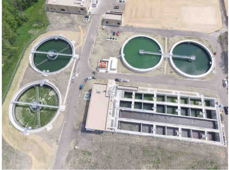
Newly Constructed Facilities for Enhanced Phosphorus Treatment at Fox Metro South Plant, Photo Credit: Fox Metro Water Reclamation District
