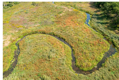
Restored North Mill Creek after Removal of North Mill Creek Dam. Photo Courtesy: Interfluve
