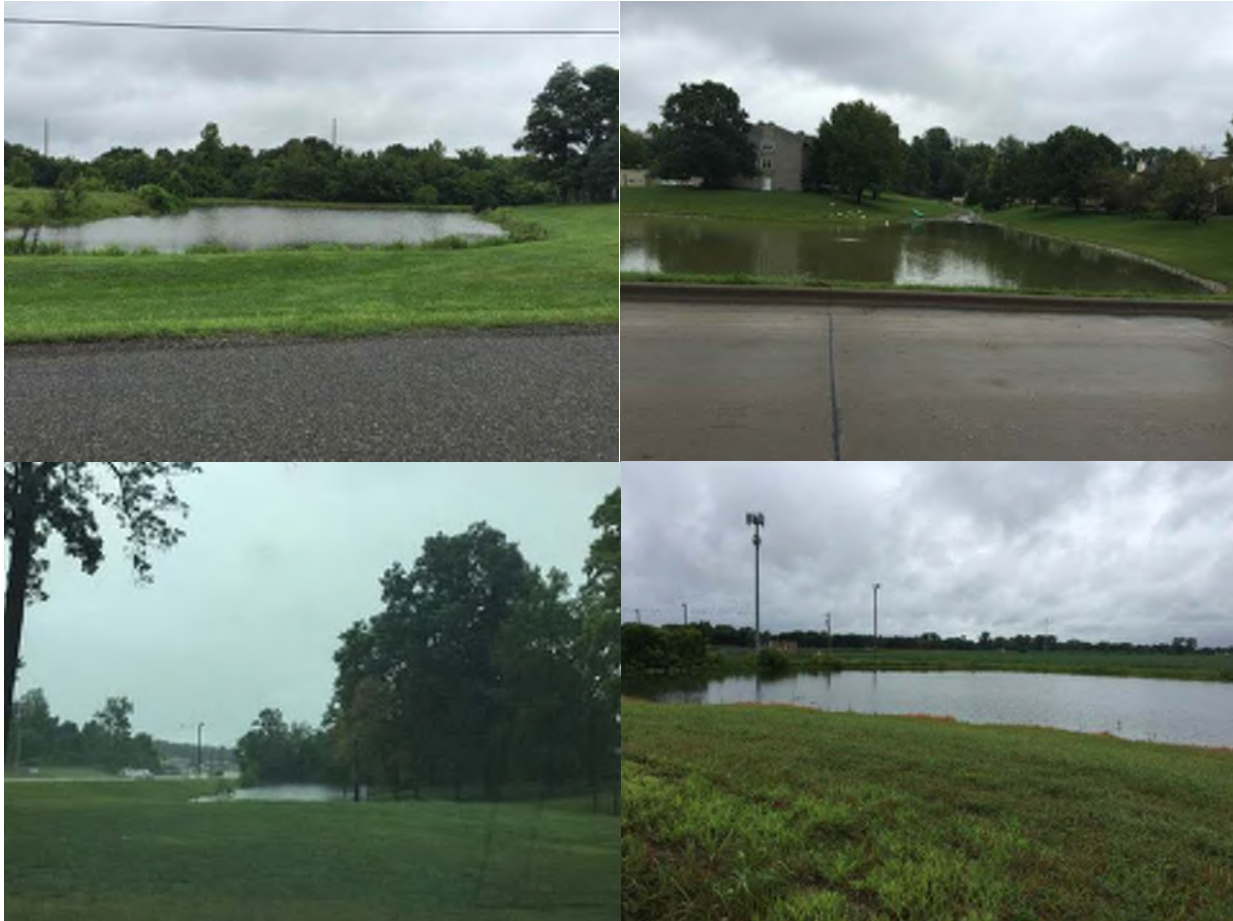
Figure A.38: Images from four detention basins from site visits on August 15, 2016. Note that Madison and St. Clair counties experienced precipitation for the past 24 hours and a flash flood warning was issued.
