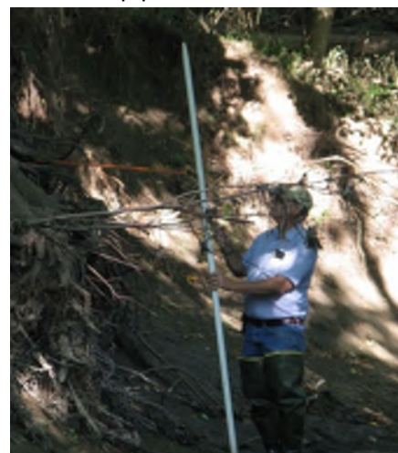
Severe streambank erosion on Silver Creek near Troy, spring 2014. Photo:HeartLands Conservancy.
