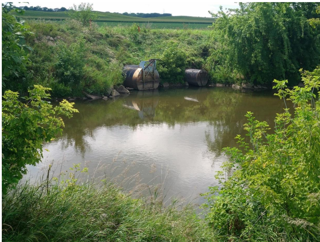
Figure 19 Drain outlet along the Green River, south of Prophetstown. Untreated discharge from fertilized fields can short-circuit denitrification zones and discharge directly into surface water.
