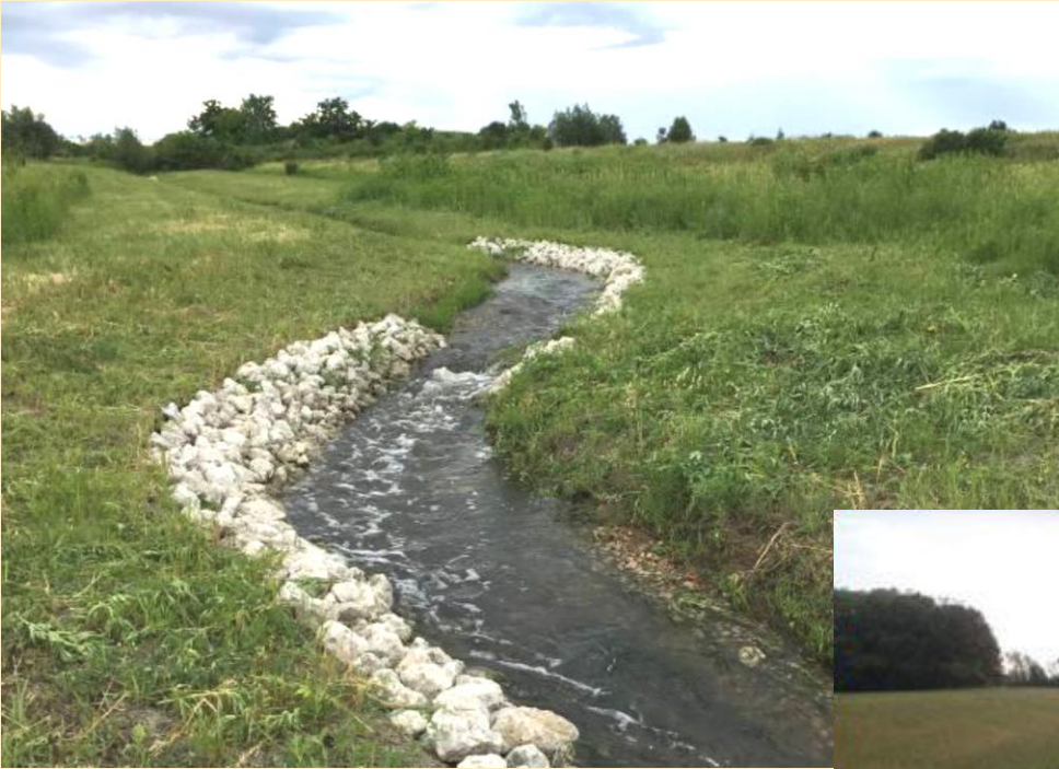
Two-stage ditch, Algonquin, IL (3191608)
