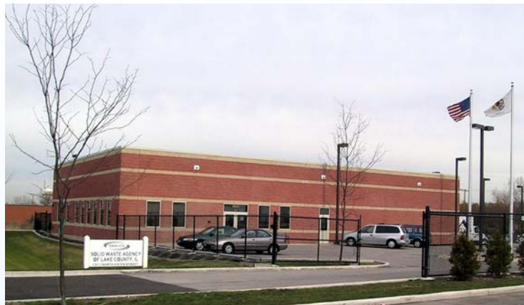
SWALCO Office and HCW Facility in Gurnee, Illinois
