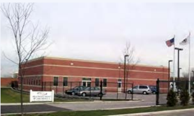
SWALCO Office and HCW Facility in Gurnee, Illinois
