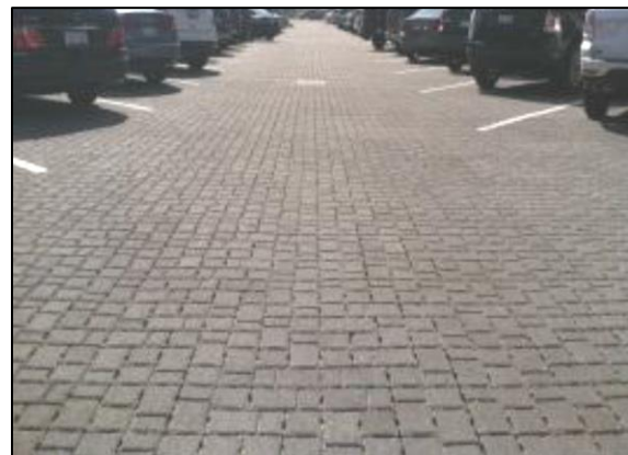
Permeable pavement parking lot post-construction.
