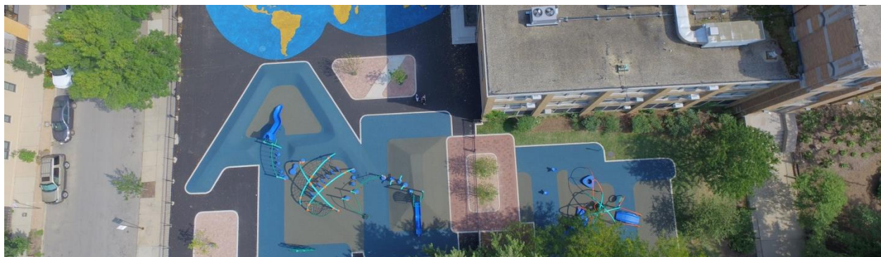
Permeable playground post-construction.
