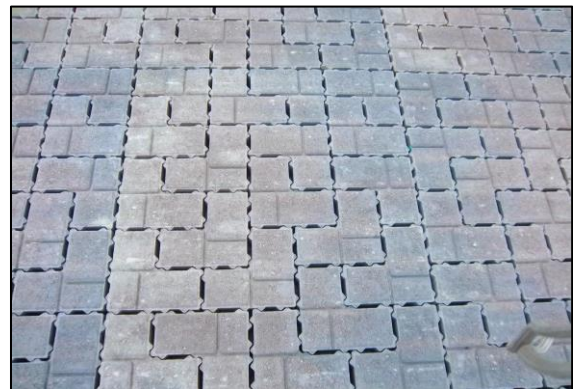
Permeable pavement alley post-construction
