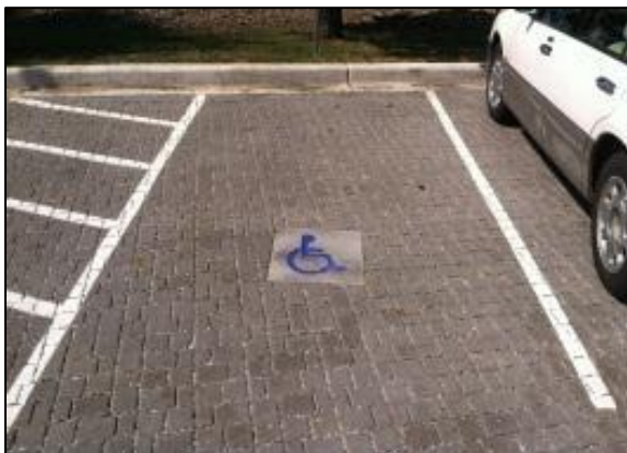
Permeable pavement parking lot post-construction.
