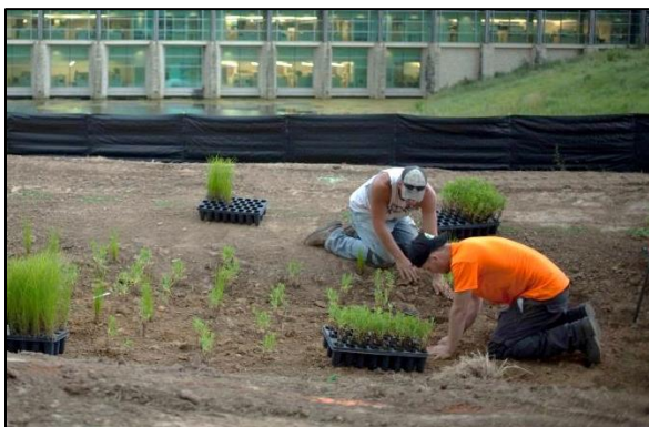
Bioswale during construction.
