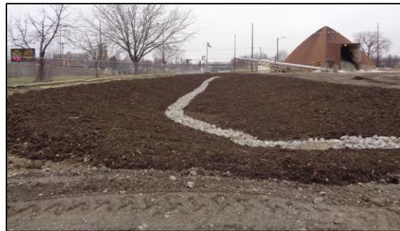
Bio-swale post-construction.
