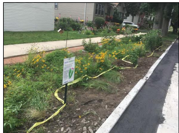
Filter of native vegetation post-construction.
