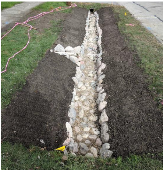
Bio-retention system during construction.
