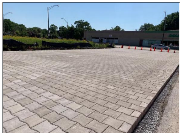
Permeable pavement parking lot post-construction.
