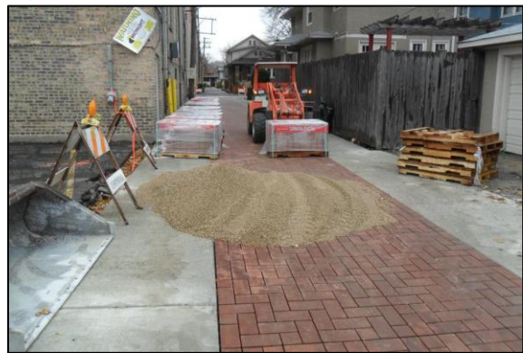
Permeable pavement alley during construction.
