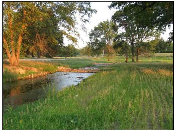
Two-stage ditch post-construction.
