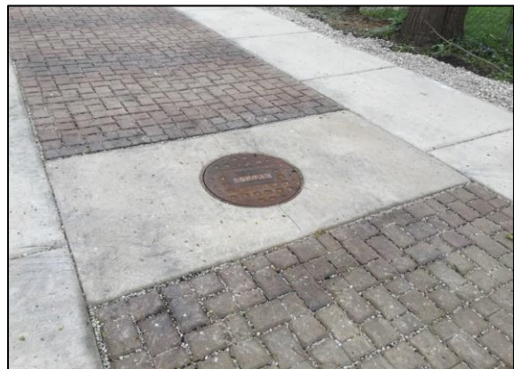
Permeable pavement alley post-construction.
