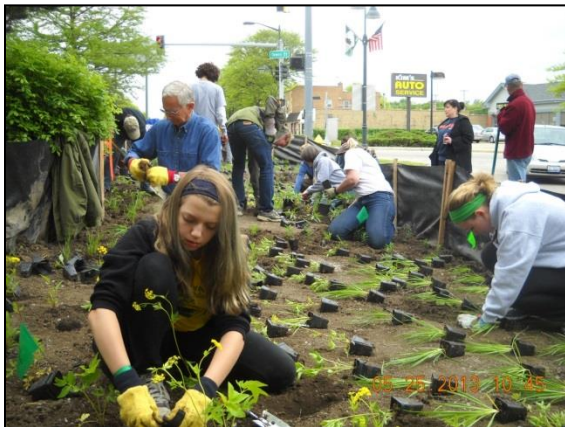
Rain garden during construction.
