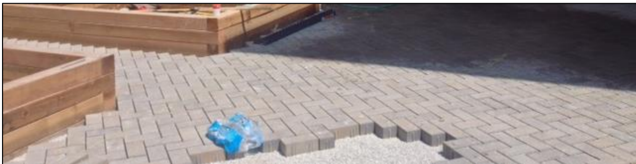
Permeable pavement during construction.
