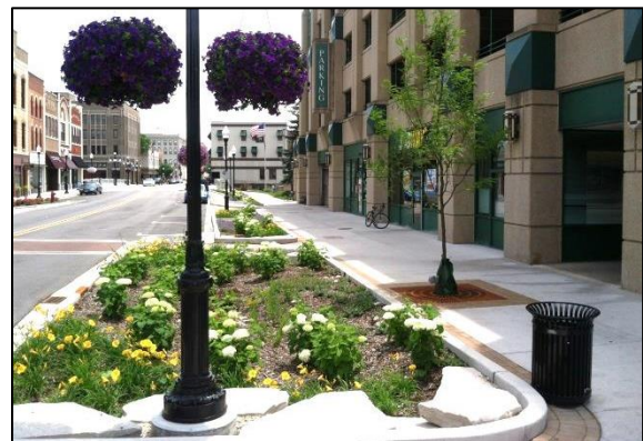
Bioinfiltration basins post construction.
