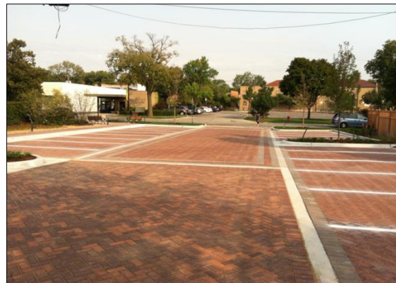
Permeable pavement parking lot post-construction.
