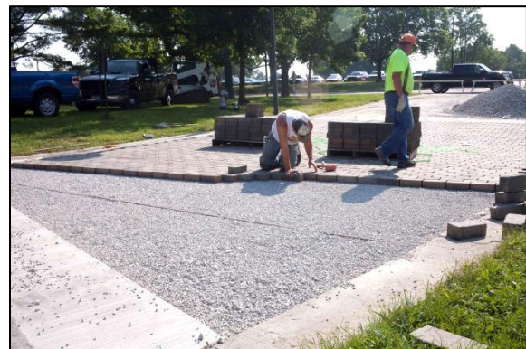
permeable pavement during construction.
