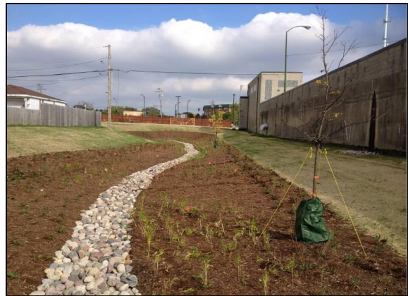
Bioinfiltration facility post-construction
