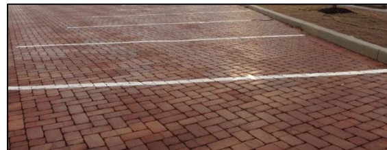
Permeable pavement parking lot post-construction.
