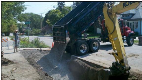
Bio-retention facility during construction.
