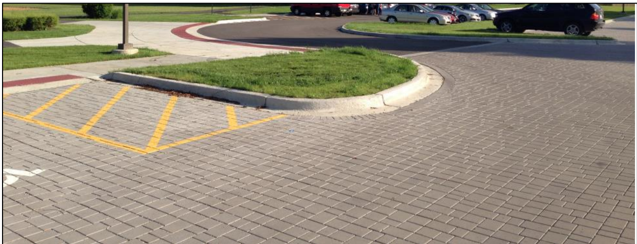
Permeable pavement parking lot post-construction.
