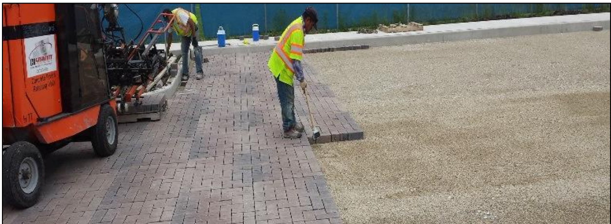
Permeable pavement parking lot during construction.
