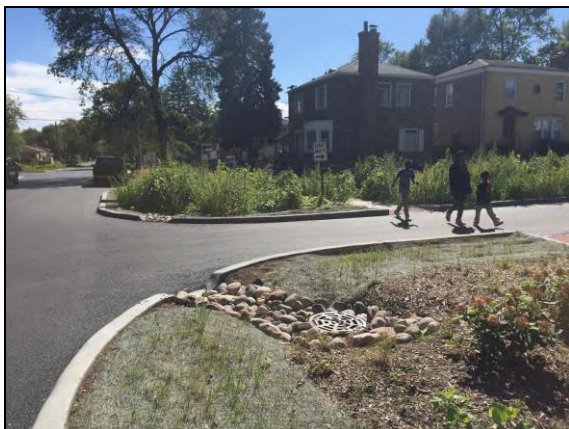
Bump-out bio-retention basins post-construction.
