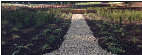
Bioswale post construction. 14-12(IGIG) SR
