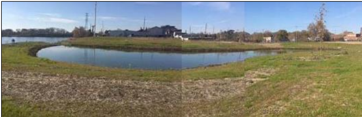
Stormwater wet pond post-construction.
