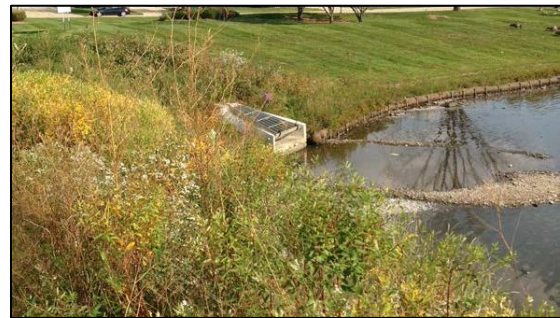
Shoreline buffer of native vegetation post-construction.
