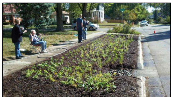
Bio-retention facility post-construction.
