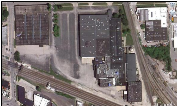
Police station site pre-construction. 12-01(IGIG) JC
