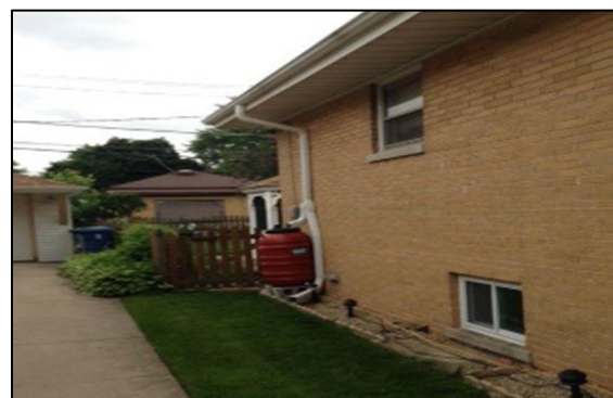
Downspout disconnection post-construction.
