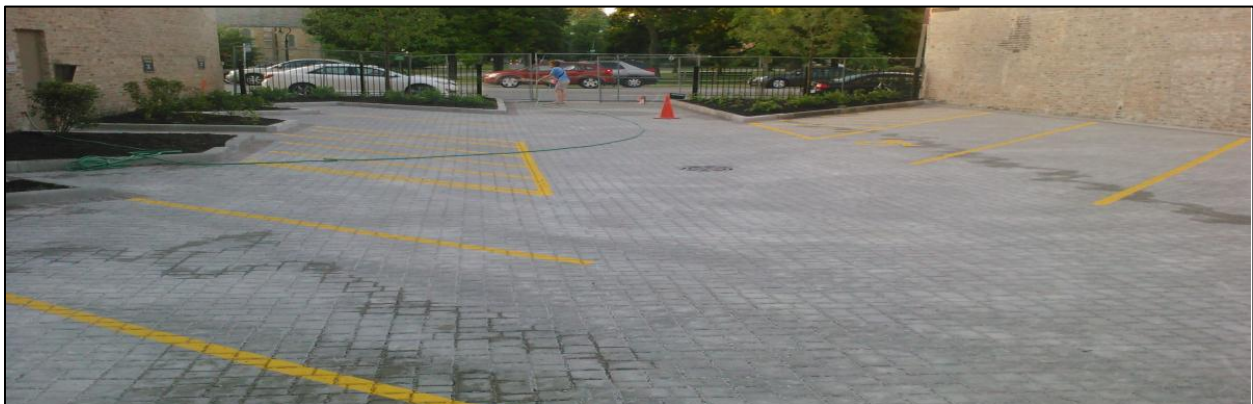
Permeable paver parking lot post-construction. 11-11 (IGIG) CD
