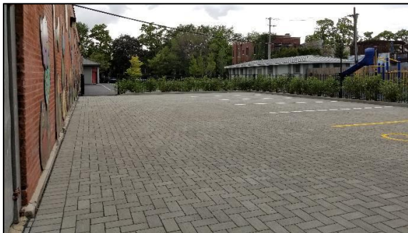
Permeable pavement parking lot post-construction.
