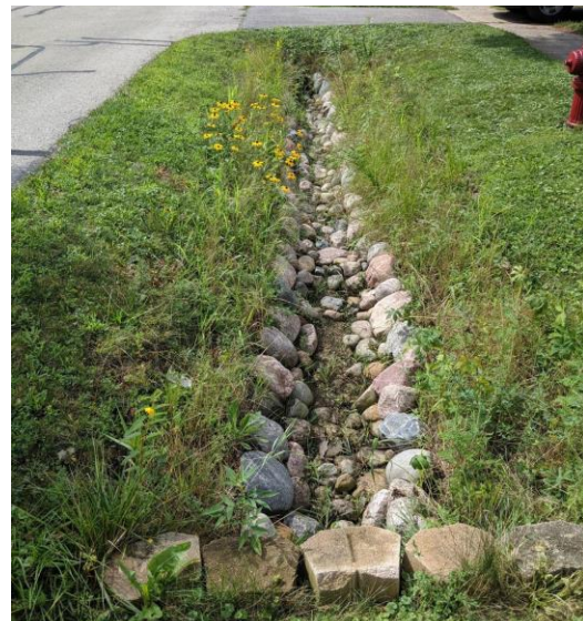
Bio-retention system post-construction.
