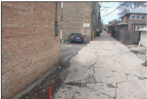
Permeable pavement alley pre-construction.
