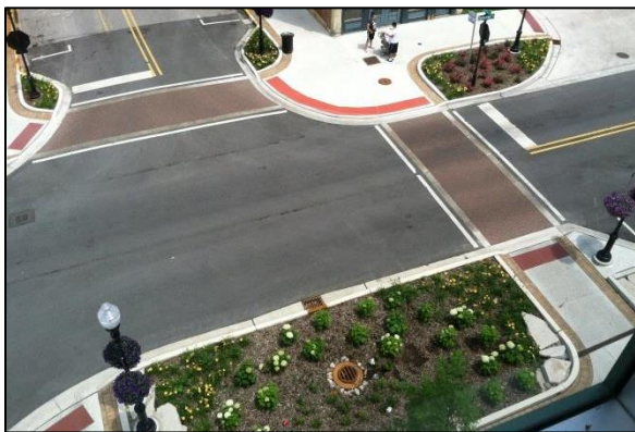
Bioinfiltration basins post construction.
