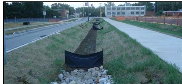
Infiltration basins post-construction.
