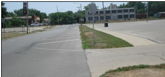
Infiltration basins pre-construction. 11-07(IGIG) SR
