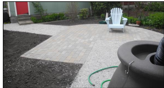
Permeable pavement & rain barrel post-construction.
