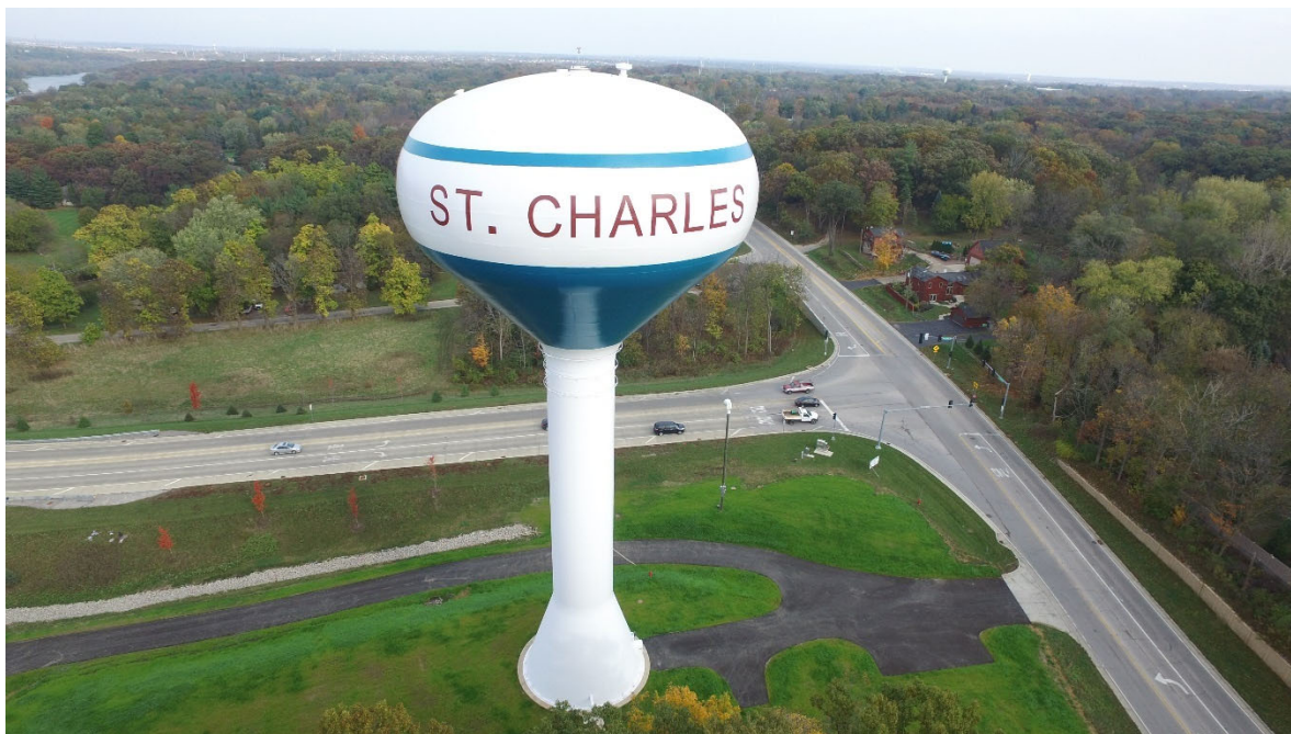
St. Charles Red Gate Road Elevated Water Storage Tank
