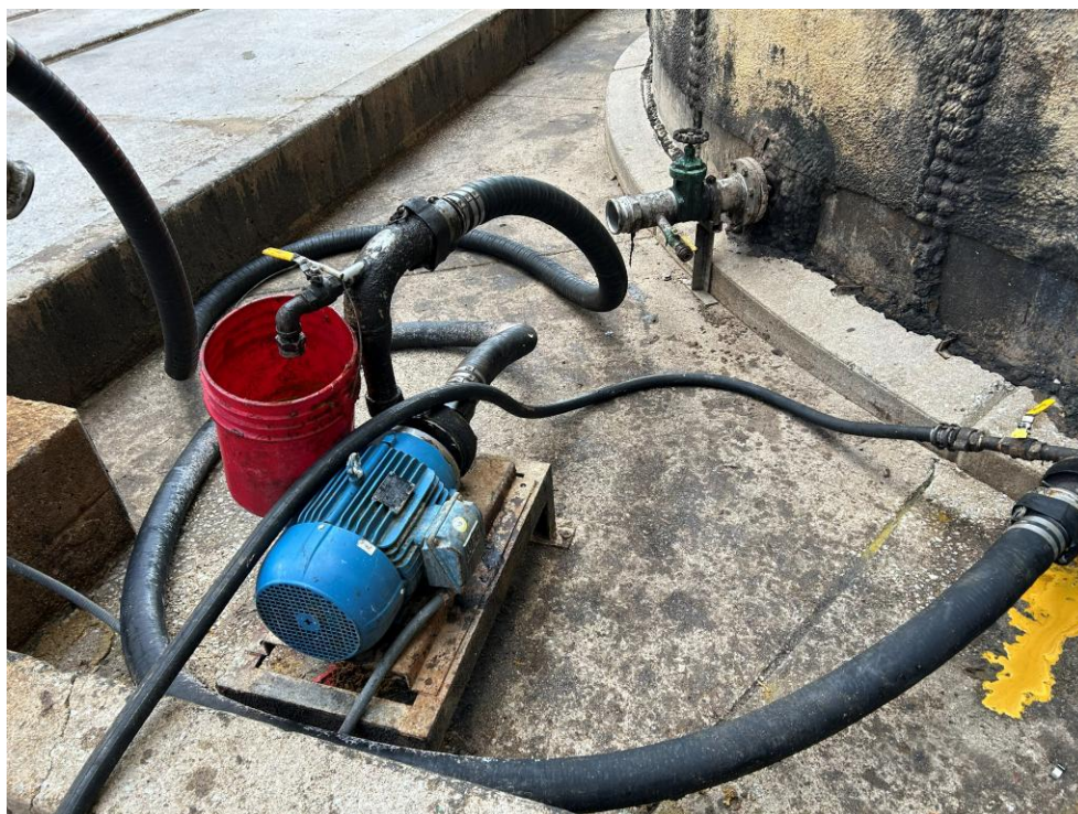
Photo 11: Connection between tanks is hoses and quick connect
