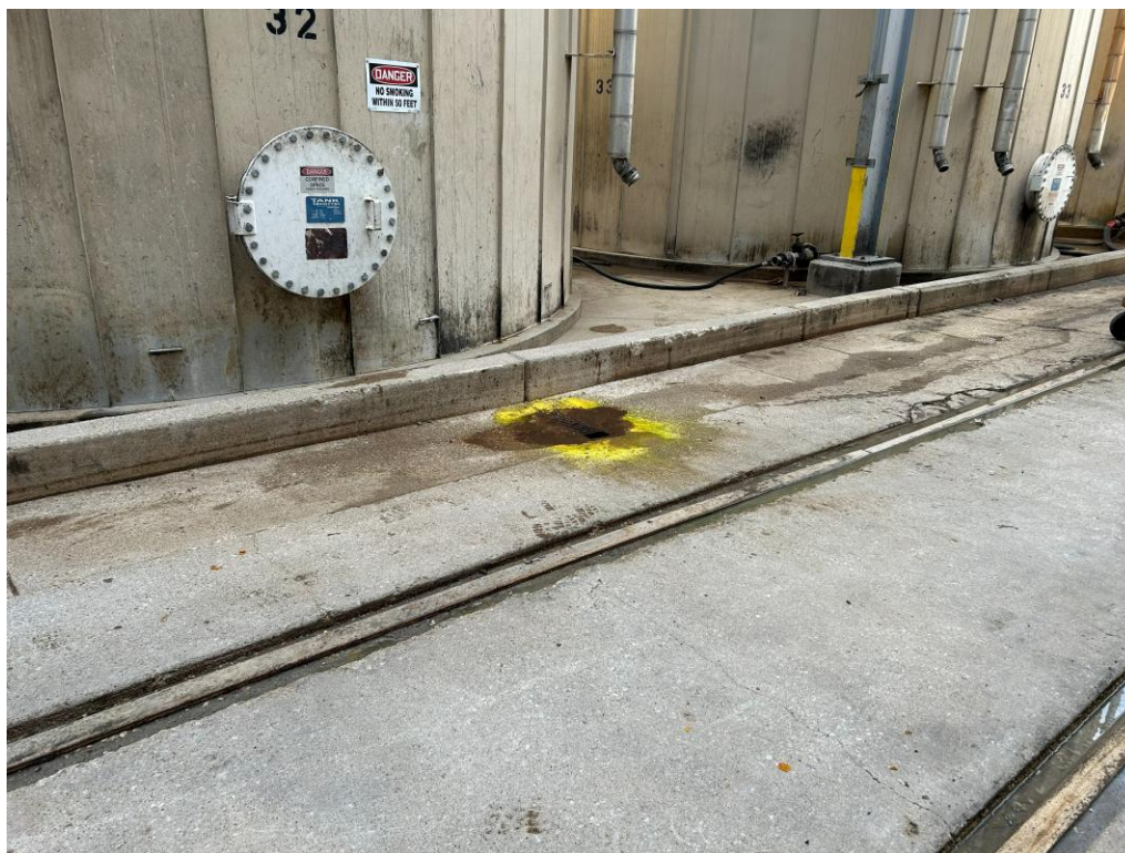
Photo 13 floor drainage, it was noted by the facility that these are underground trenches
