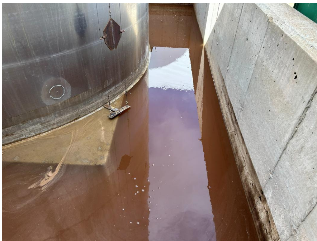
Photo 4: inside the dike area of Sludge tank T47
