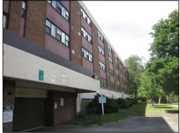
2. Another view of the Fox Shore building
