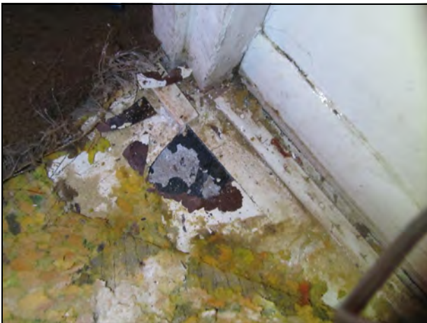
27. Close-up of the previous photo.
