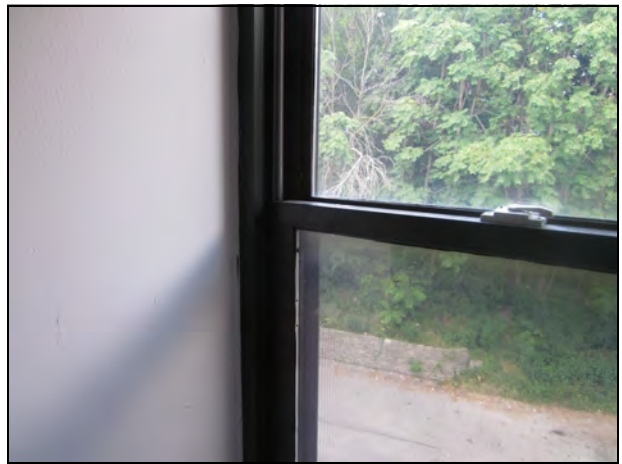
34. View of a typical window with caulk.
