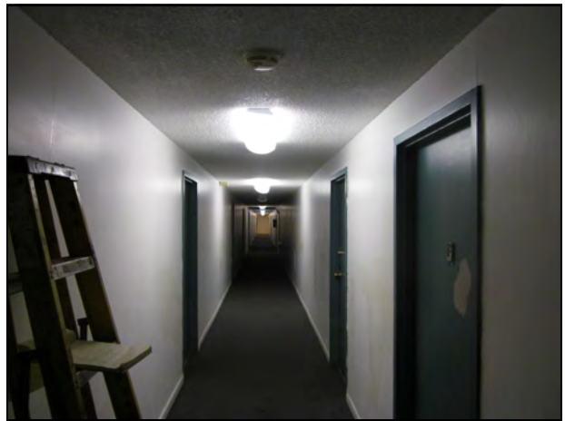
16. View of a typical common hallway.
