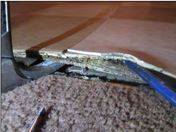
29. Close-up of the previous photo.
