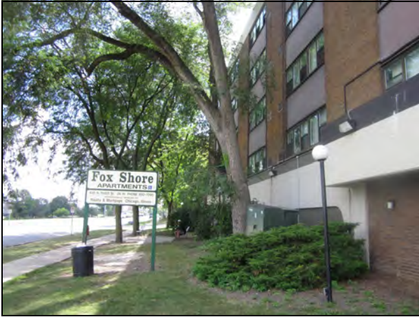
1. View of the Fox Shore building.
