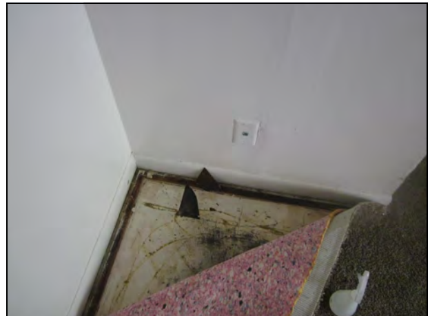
24. Another view of the same flooring system present in another unit.
