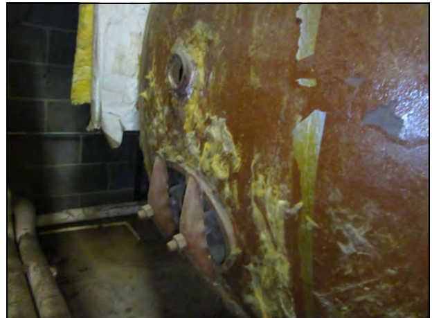
6. Close-up of the previous photo.
