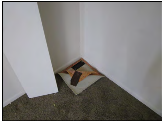
22. View of a bedroom closet; the pulled back carpet reveals floor tile and black mastic.
