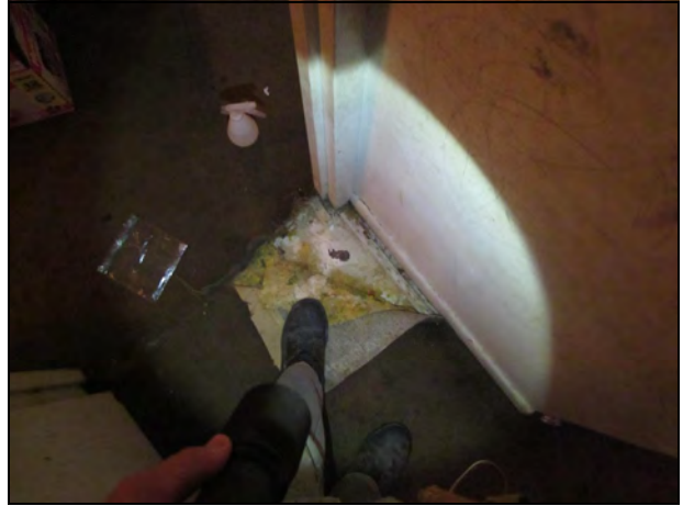
26. Another view of the same flooring system.
