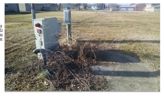
Photo #011Date:February 25, 2021Time:8:46 a m.Taken By:Joe Stitely, BOWFacility:Commonfields of CahokiaLocation:53<sup>rd</sup> & Market Station (#3)Notes:This is a photograph of the<br/>sewage debris on the<br/>ground surface adjacent to<br/>the lift station.
