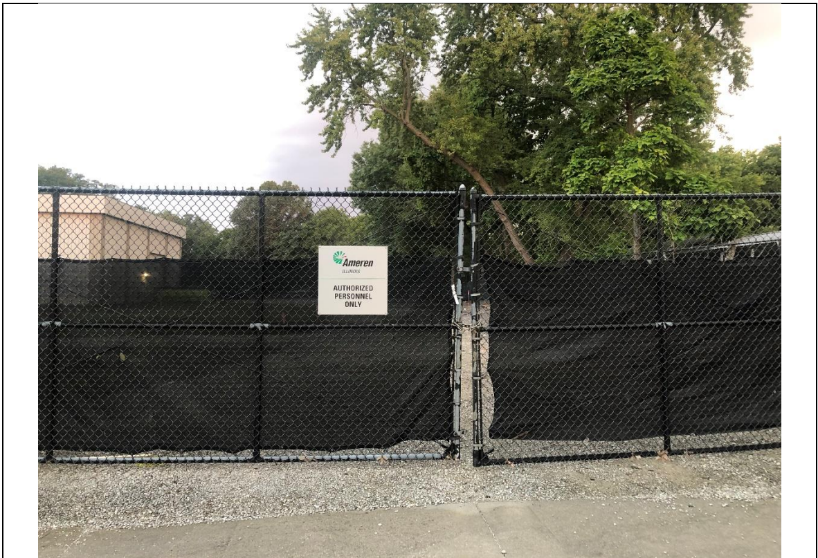
Photograph 1 North gate to Site with fencing and signage, looking west.
