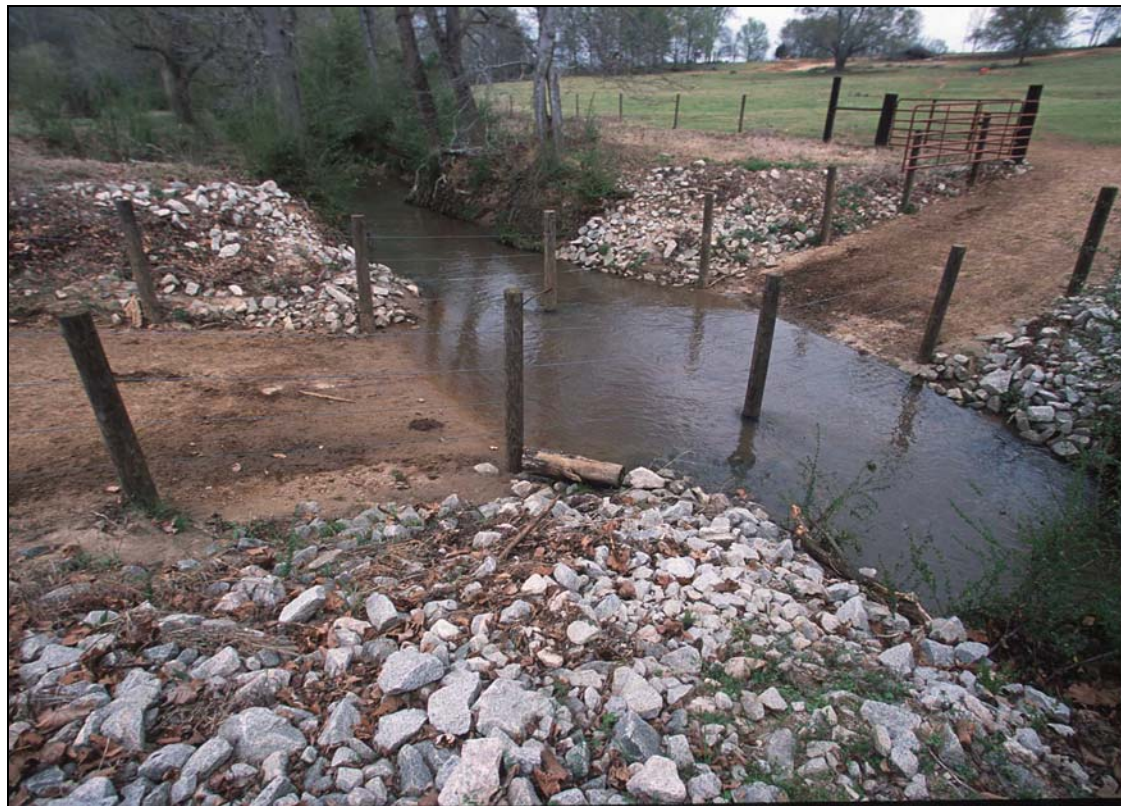
Figure 4-13. Restricted Cattle Access Point with Reinforced Banks.
