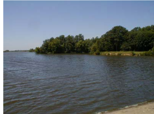
Vandalia Lake at Illinois Rt. 15 crossing, looking southwest at bank erosion.
