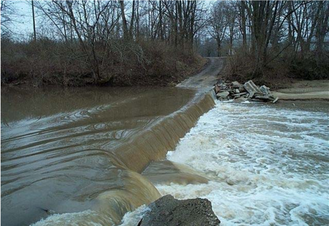
Fig. 15 Low water crossing on Rd. S625 with 3-4 ft. overfall (Chapter 2)
