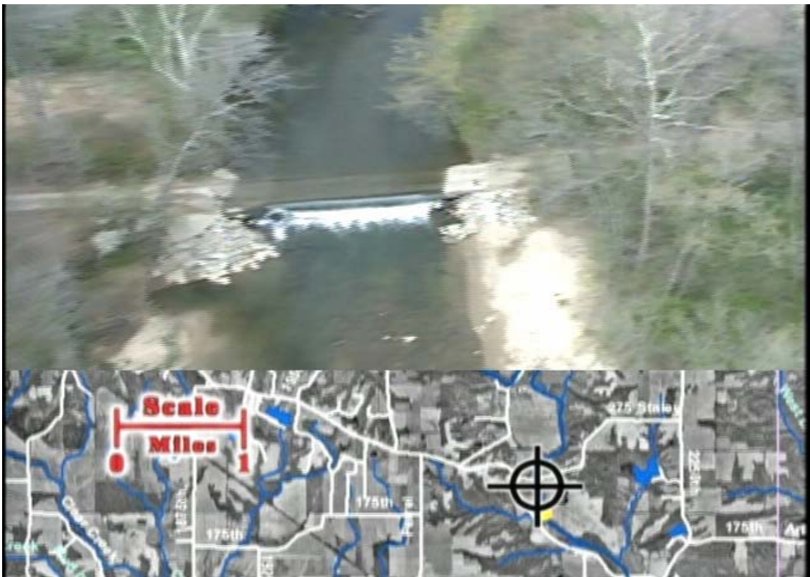
Fig. 8 Concrete ford with 3-4 ft. overfall on Road S625
