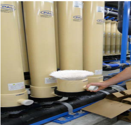
Figure 15. Macomb water plant hollow fibers inside PALL filter modules
