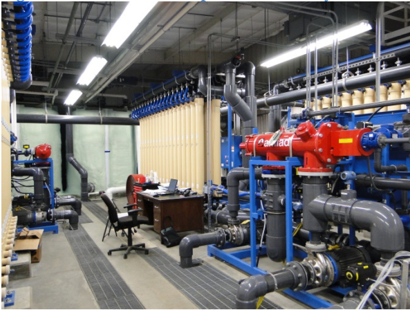
Figure 15. Macomb water plant hollow fibers inside PALL filter modules
