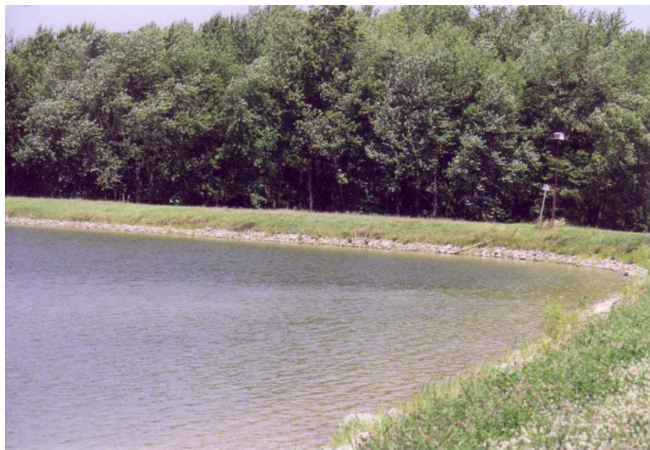
Wayne City Side Channel Reservoir (Segment RCT)
