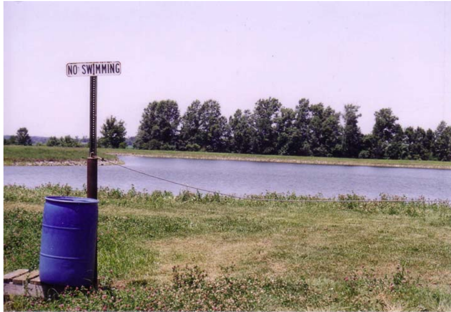
Wayne City Side Channel Reservoir (Segment RCT)
