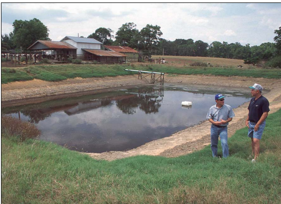
Figure 4-6. Waste Storage Lagoon.
