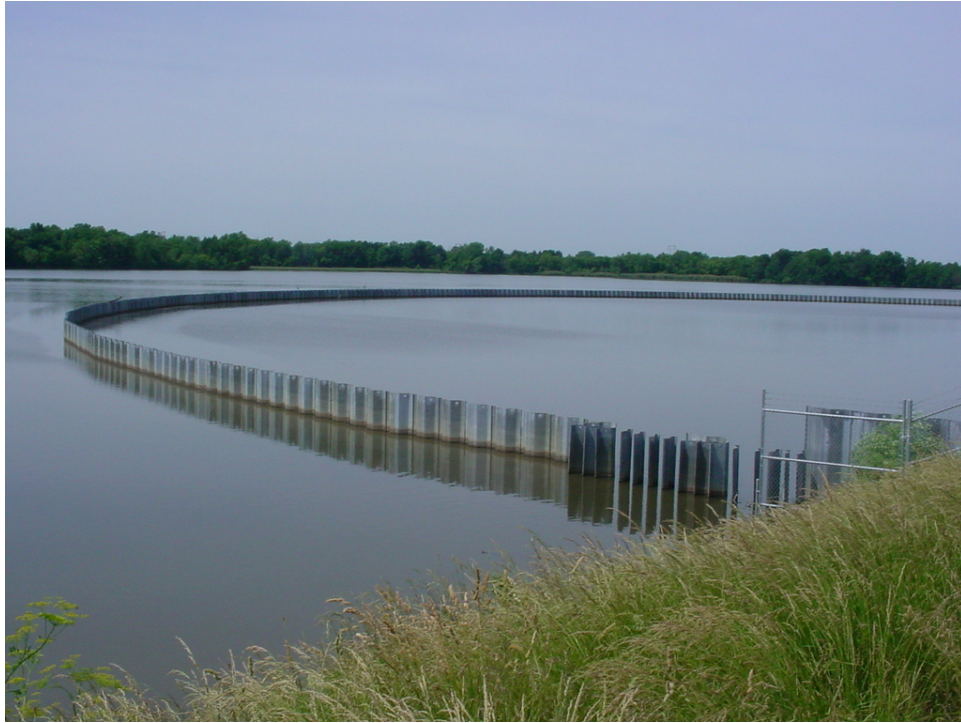
Lake Taylorville: Sediment Retention Structure
