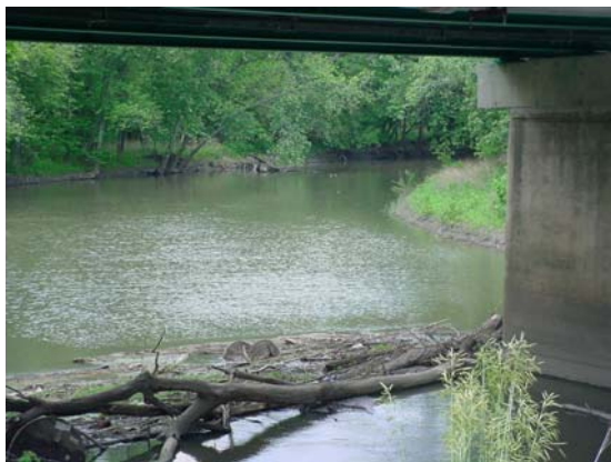
Sangamon River Segment E29 at Route 136 Looking Northeast
