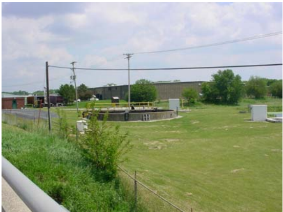
Fisher Sanitary Treatment Plant
