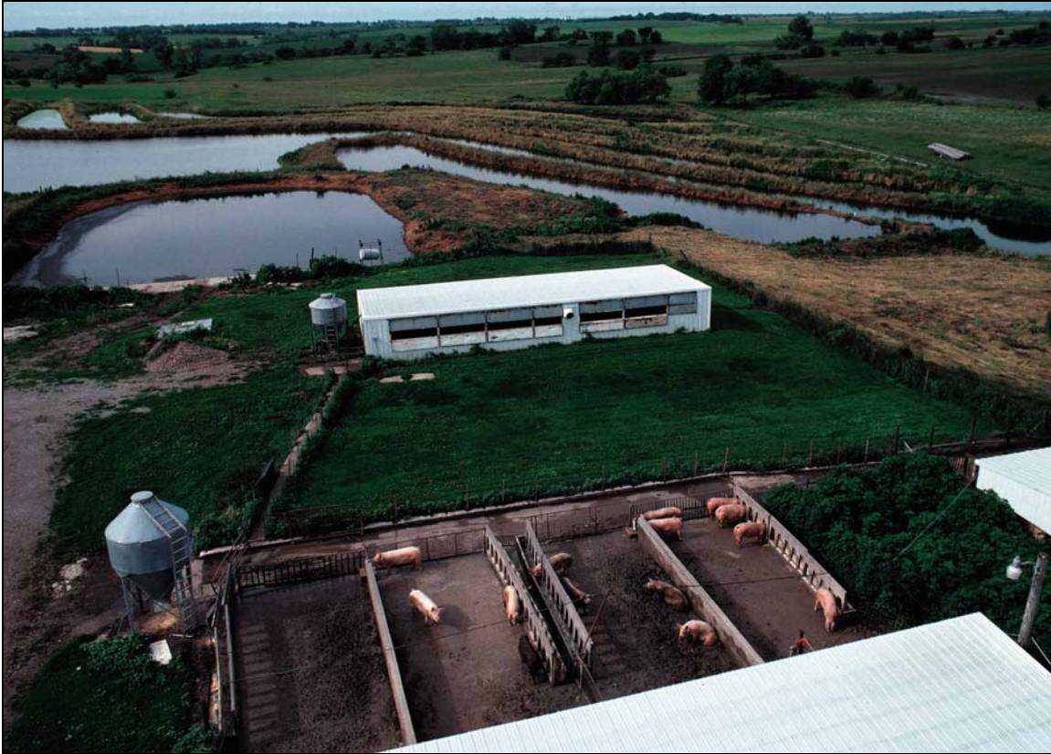
Figure 5-9. Constructed Wetland System for Animal Waste Treatment.
